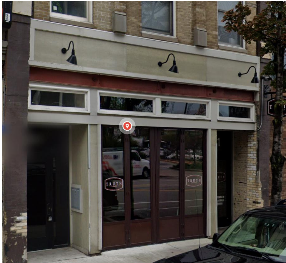
Current appearance, guard will go in front of accordion door.
