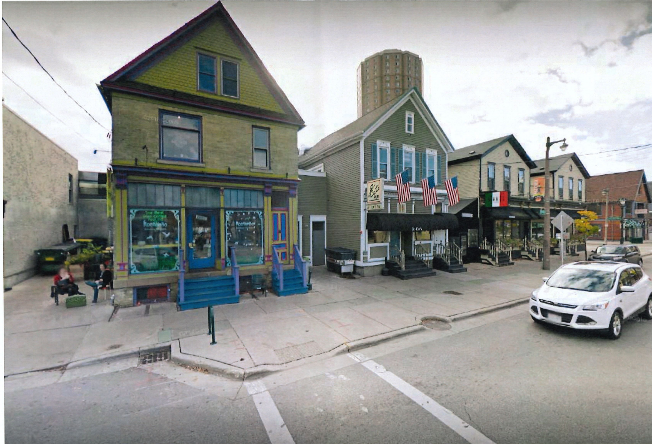
STREET VIEW - FROM NORTH-EAST
