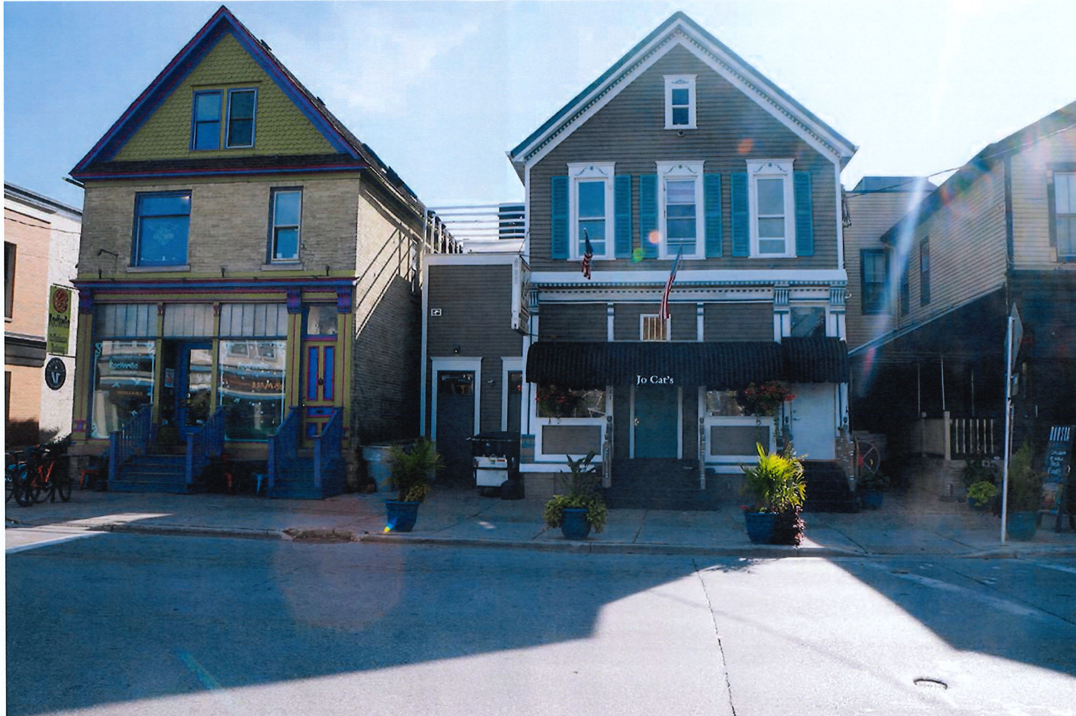
STREET VIEW - FROM NORTH
