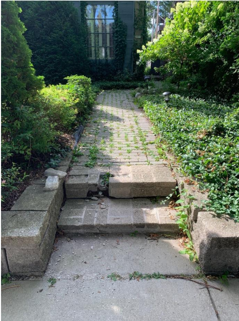
Current condition of the front walk – crumbling pavers, missing pavers, leaning retaining walls
