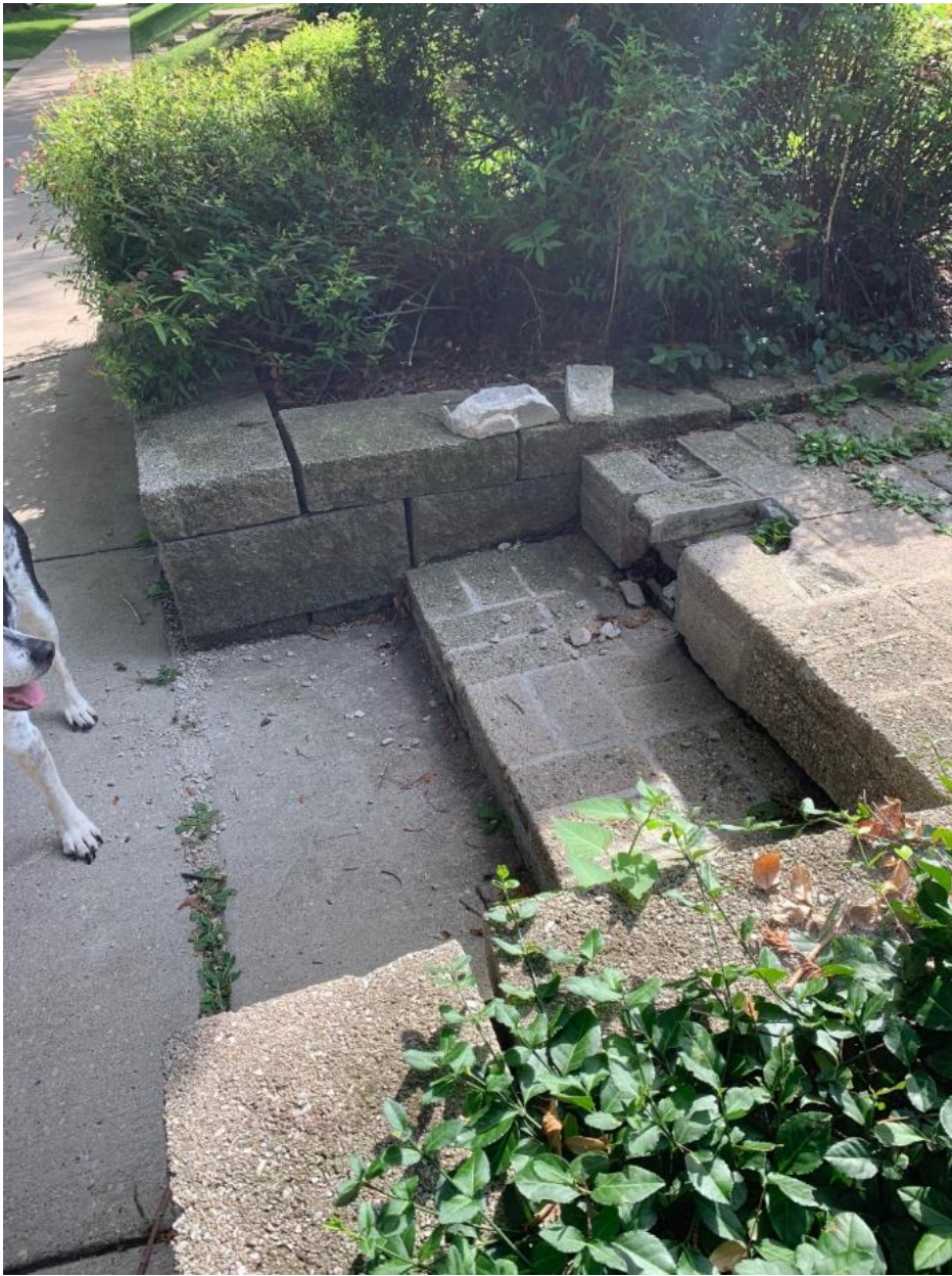
Current condition of the front and side walk – crumbling pavers, missing pavers, leaning retaining walls
