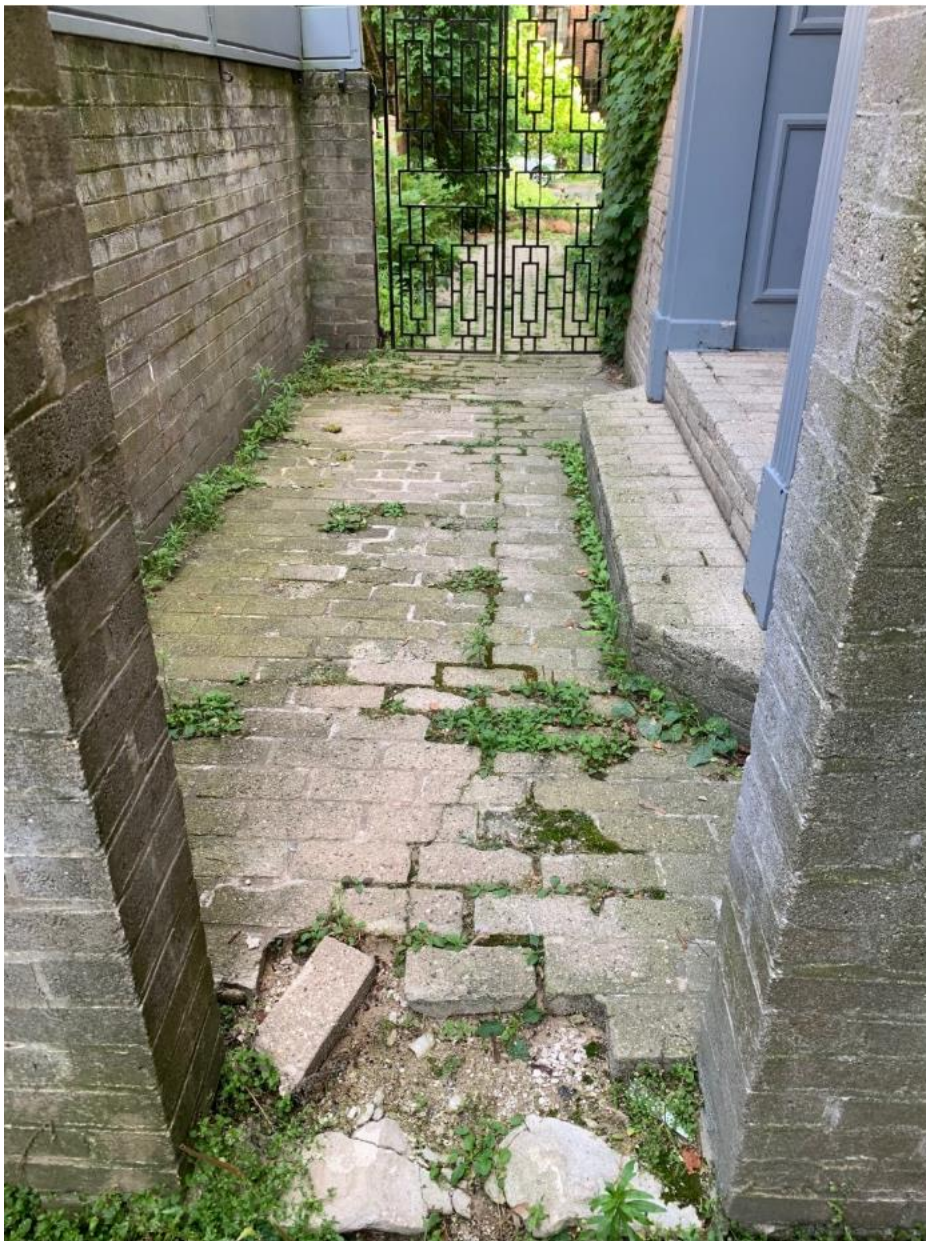
Current condition of the side walk – crumbling pavers, missing pavers, existing arborvitae hedge to be removed
