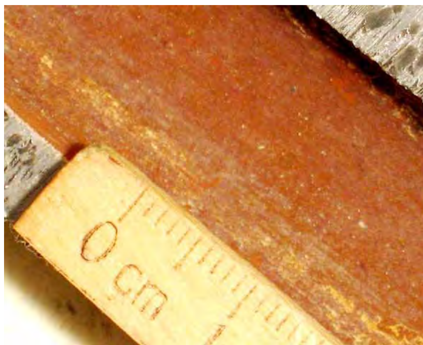
Figure F.41 Photograph of Pipe PP06 from Site D2
