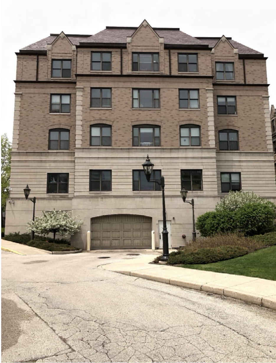
Watertower East elevation – Lake Dr
