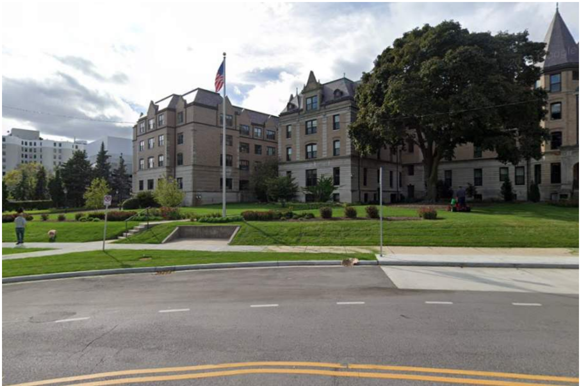
Watertower – Northeast View from Downer Ave Public Way
