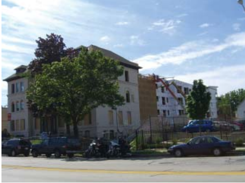
Empowerment Village is building a major addition to an existing building.
