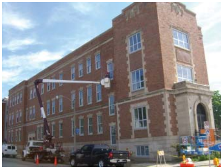
Sometimes existing buildings can be adaptively reused - Johnston Center.
