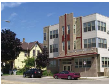
The recently developed Prairie Apartments
