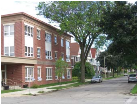
United House fit nicely into the neighborhood.
