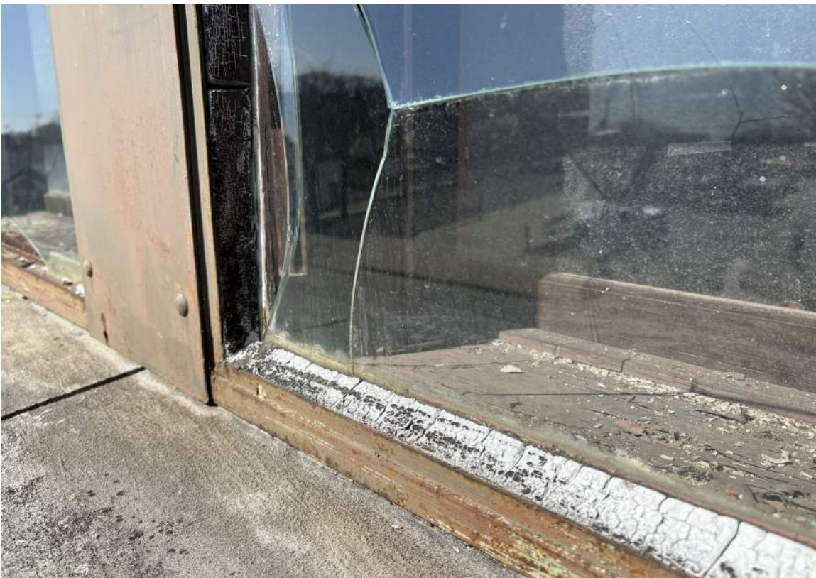
IMAGE 41: Exterior - looking down at sill frame of original steel sash window with broken glass and beveled glazing putty (photo from boom lift)
