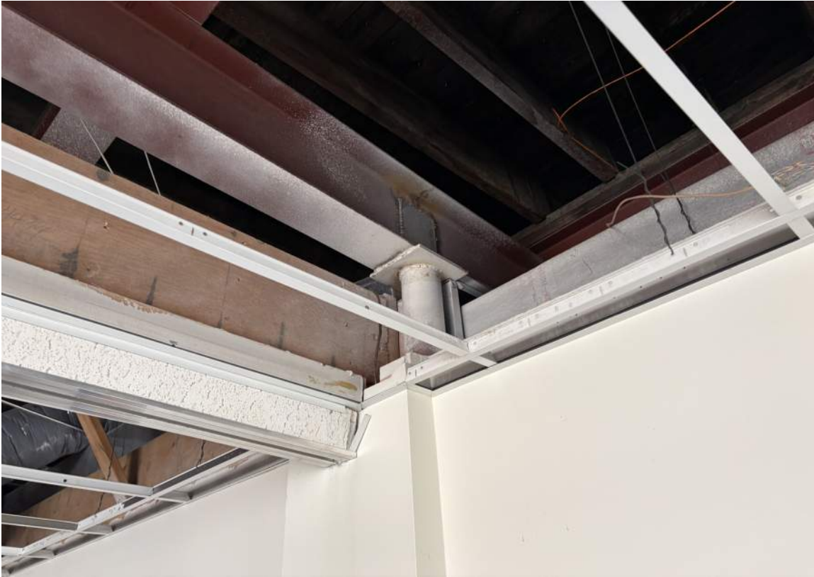
IMAGE 142: Level 02 - 1891 Structure - looking southwest and up at existing tube steel column and steel beam overhead below wood roof framing
