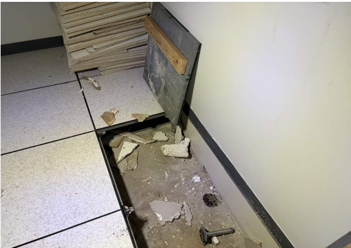
IMAGE 111: Level 02 - 1949 Structure - looking down at removed portions of raised floor system over concrete floor
