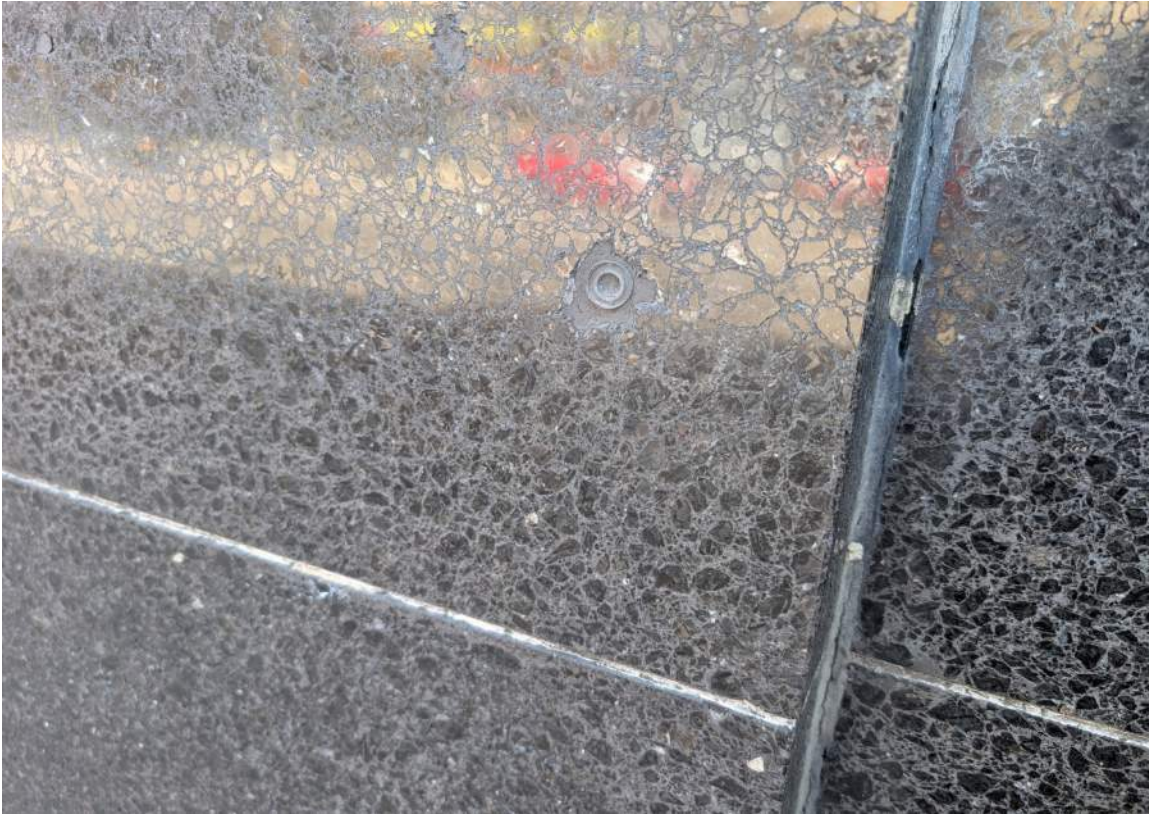
IMAGE 14: Exterior - cast granite panels with existing penetration and signage anchor
