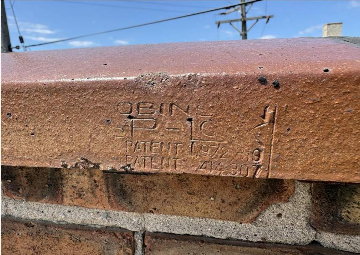
IMAGE 168: Rooftop - 1949 Structure - close up of existing clay tile parapet caps
