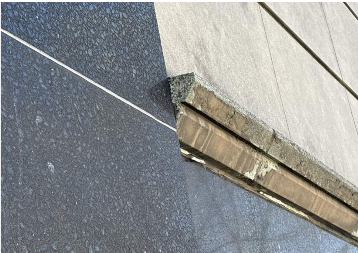
IMAGE 10: Exterior - looking up at close up view of existing cast granite panels, limestone belt course, and cut limestone (photo from boom lift)
