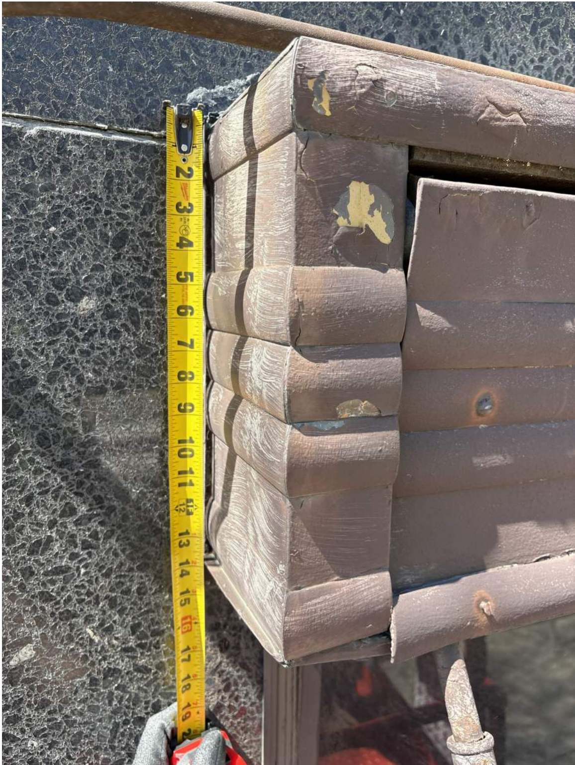
IMAGE 29: Exterior - close up photo of end cap on existing fluted bronze storefront headed (photo from boom lift)
