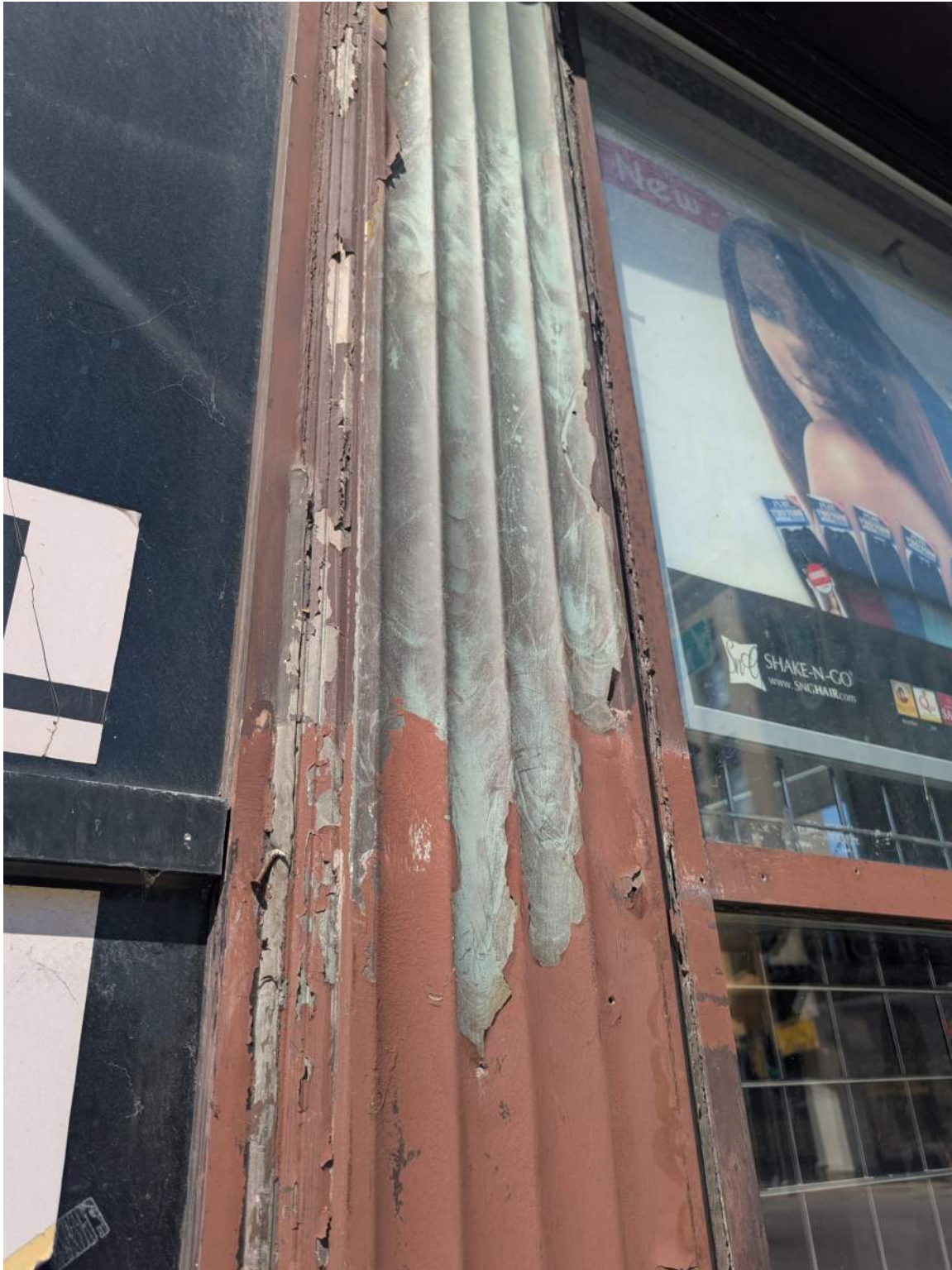
IMAGE 22: Exterior - looking up at bronze fluted mullion with flaking paint and existing storefront system with perimeter trims
