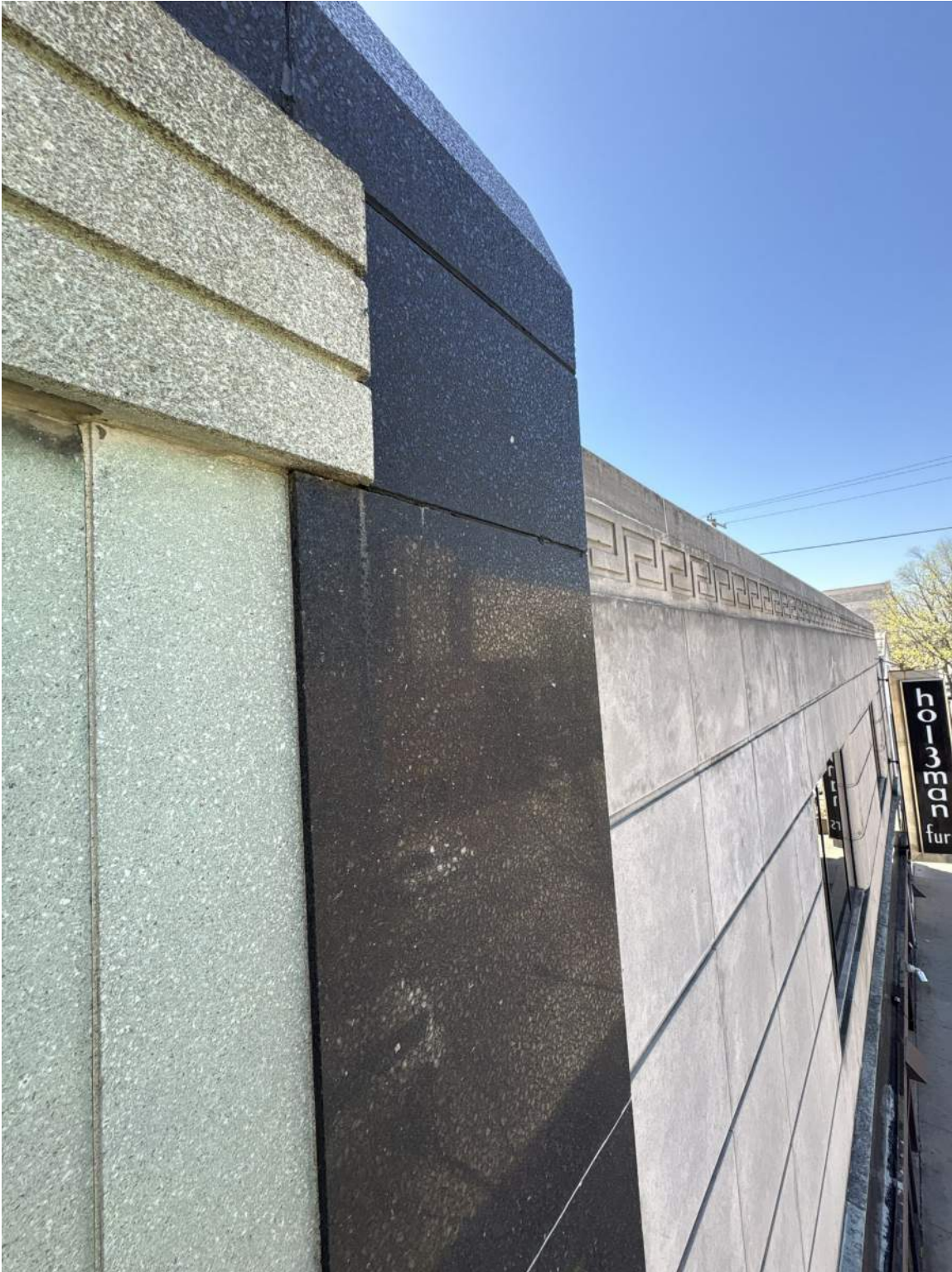
IMAGE 13: Exterior - looking east at cast granite panels and cut limestone at stepped rooftop condition (photo from boom lift)
