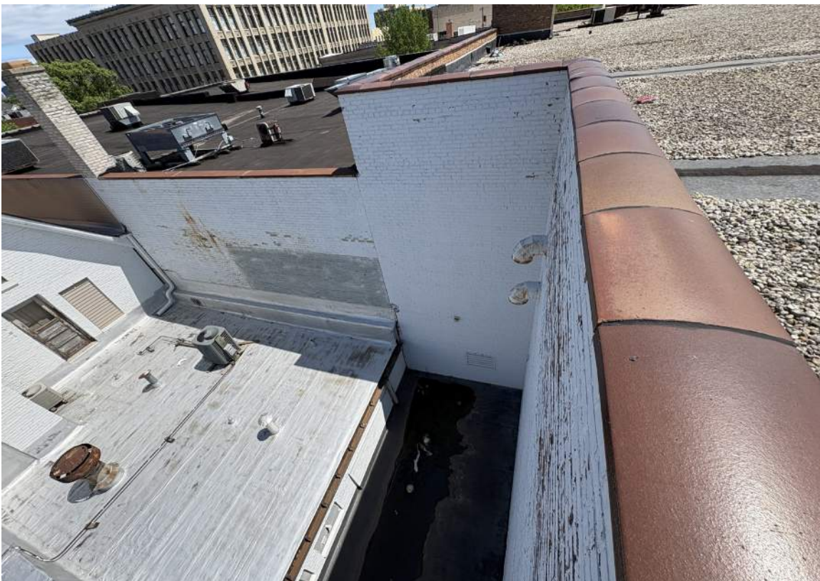
IMAGE 167: Rooftop - 1949 Structure - looking northeast at clay tile parapet caps and abutting neighboring building below
