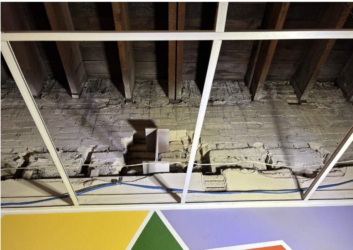
IMAGE 145: Level 02 - pre-1888 Structure - looking up and east at masonry walls separating in 1891 Structure with penetrating steel beam
