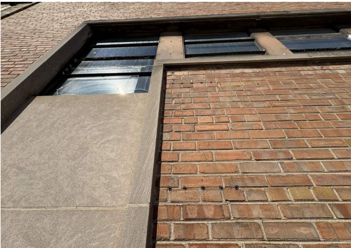
IMAGE 43: Exterior - looking up at original projecting limestone accents and wall cladding above stair exit door
