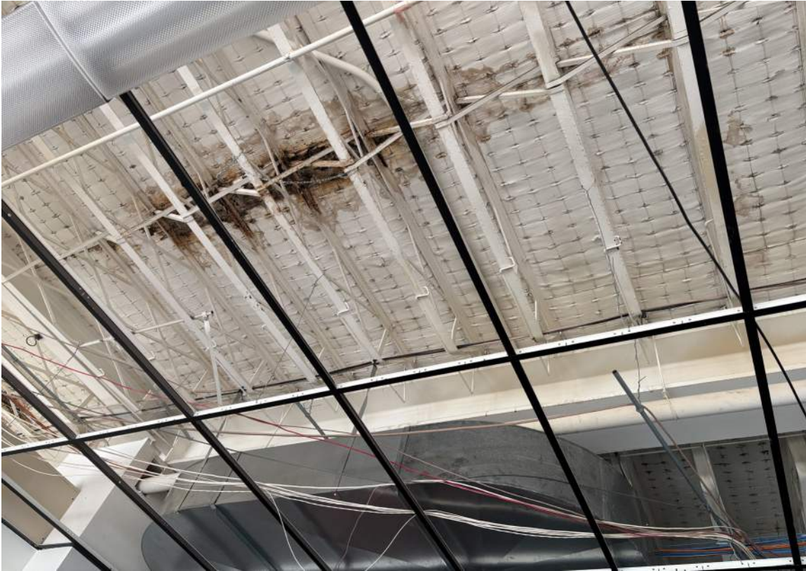
IMAGE 112: Level 02 - 1949 Structure - looking up at water infiltration and rust at existing steel roof joists
