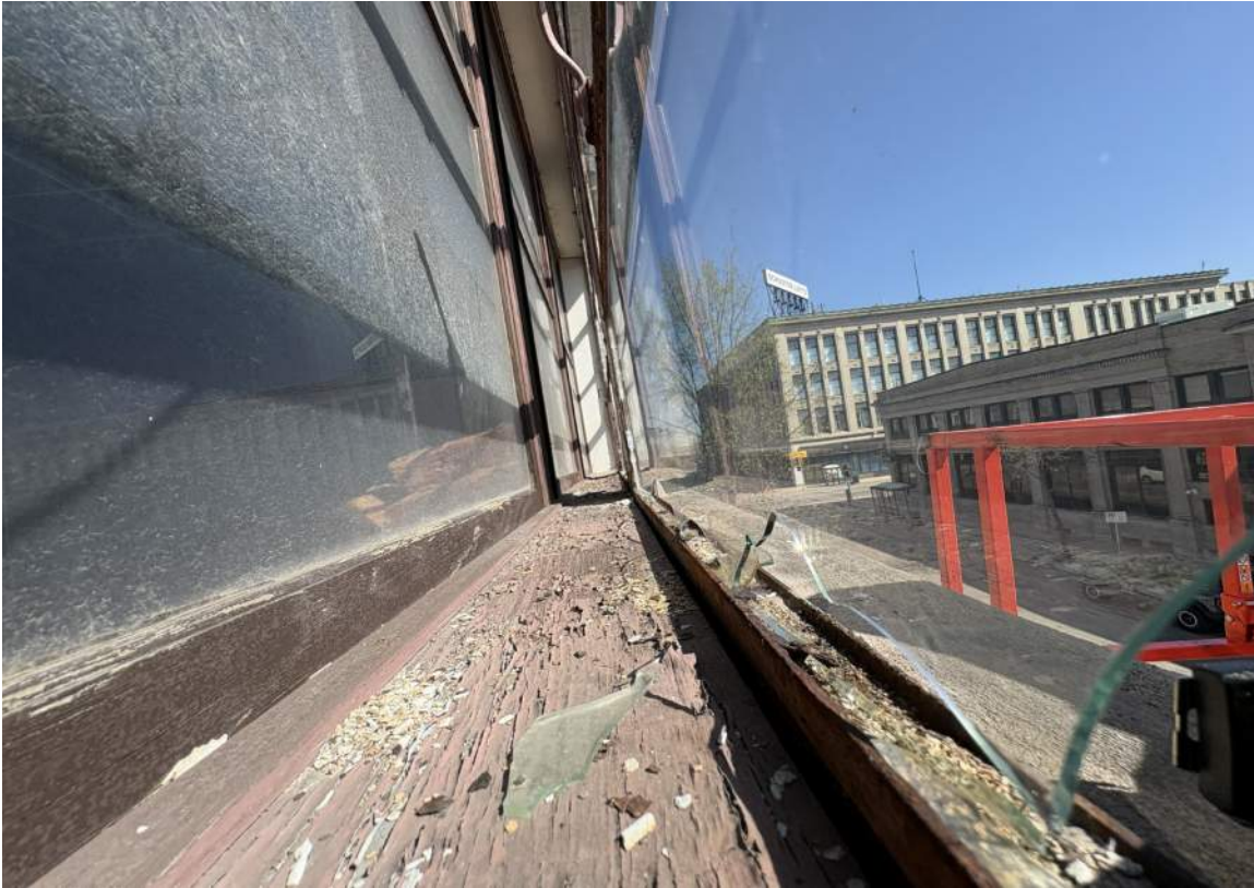
IMAGE 42: Exterior - looking north - inside original steel sash window is on the righthand side and original wood storm windows is on the lefthand side (photo from boom lift)
