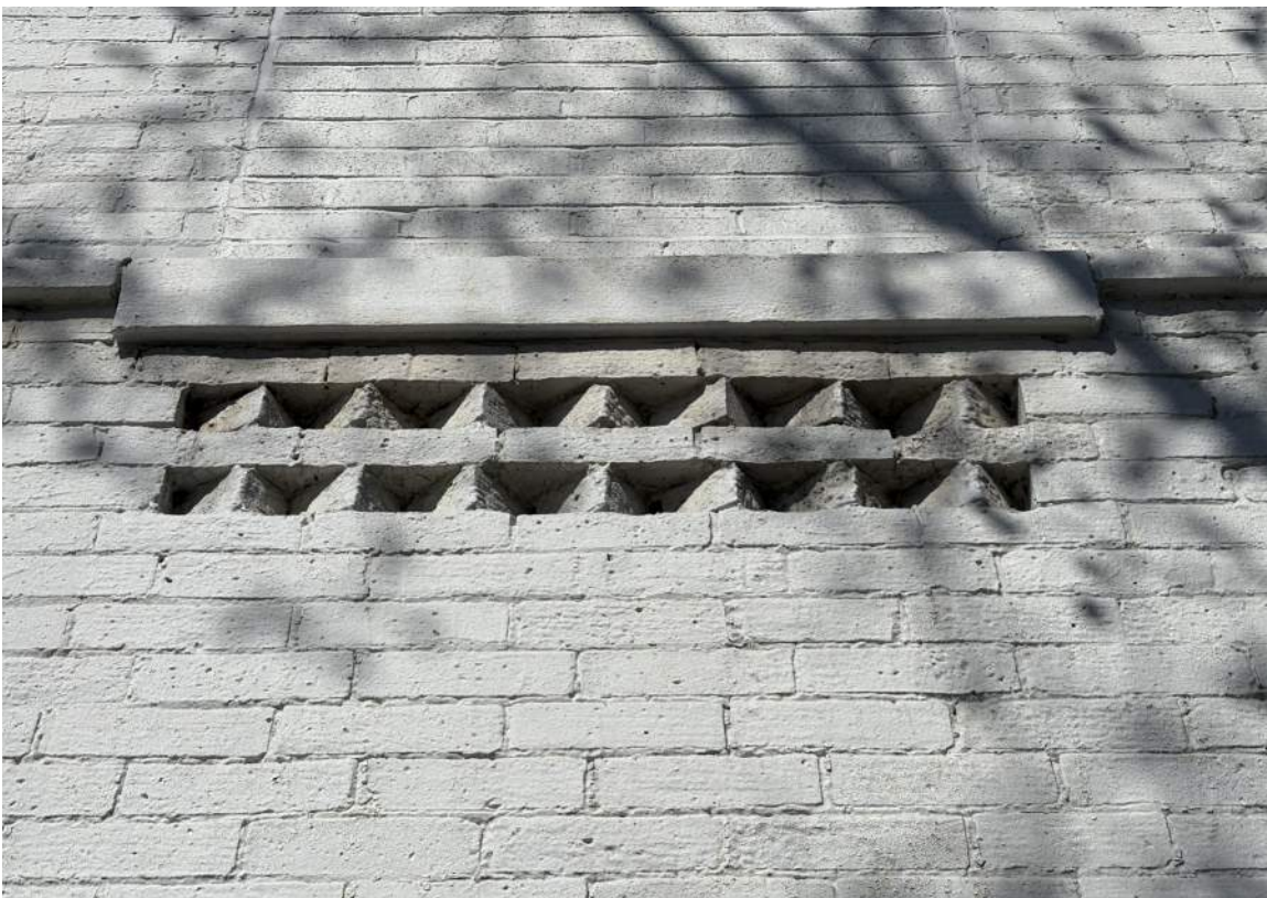
IMAGE 35: Exterior - looking up at existing brick infilled opening with remaining limestone sill and original rotated brick vents below
