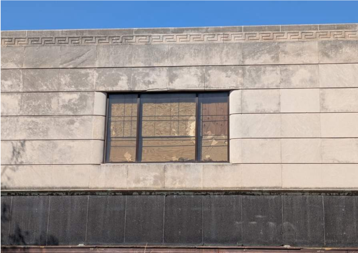
IMAGE 25: Exterior - looking west at existing storefront window in cut limestone facade; split limestone header above window head
