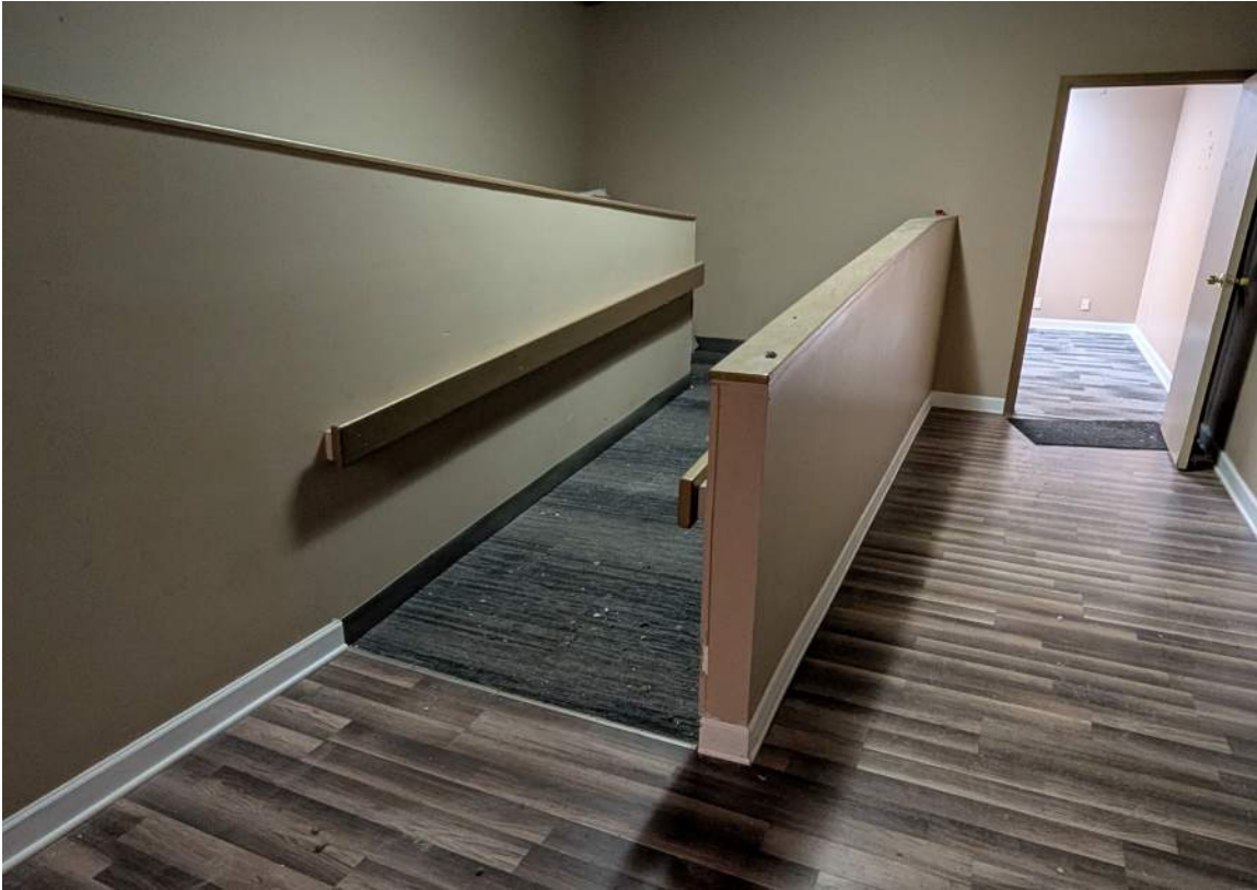
IMAGE 133: Level 02 - 1911 Structure - looking northwest at existing overframed ramp
