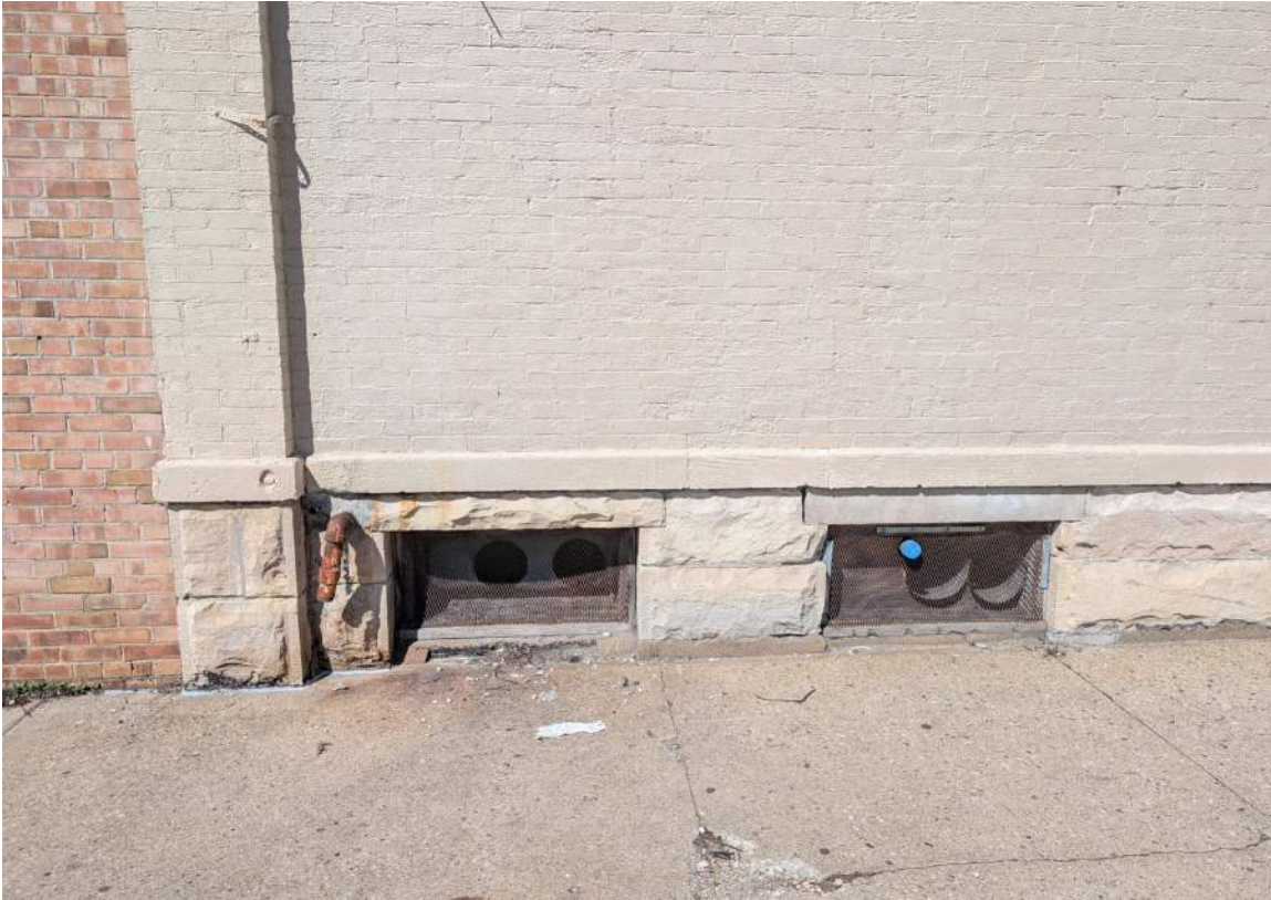
IMAGE 32: Exterior - looking west at brick and rusticated stone wall with existing openings to basement; right hand existing lintel has already been replaced
