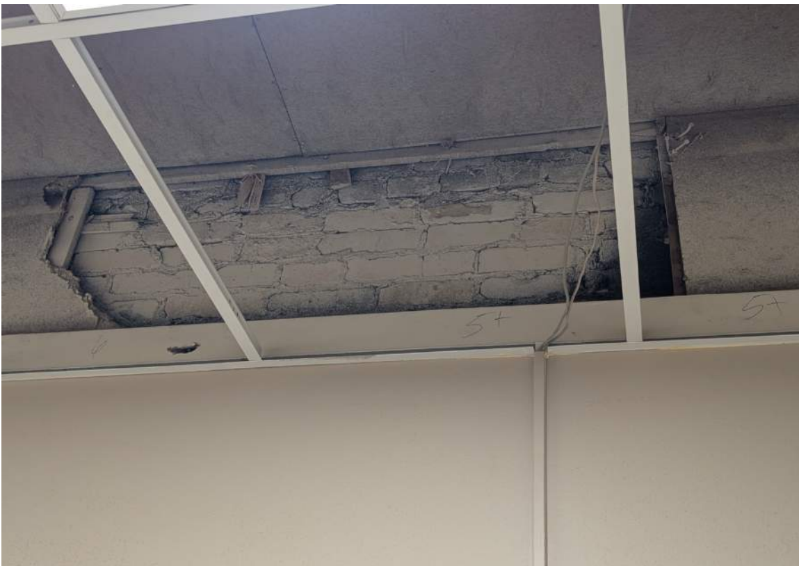
IMAGE 159: Level 02 - pre-1888 Structure - looking west and up at small portion of brick masonry wall exposed above existing wall furring
