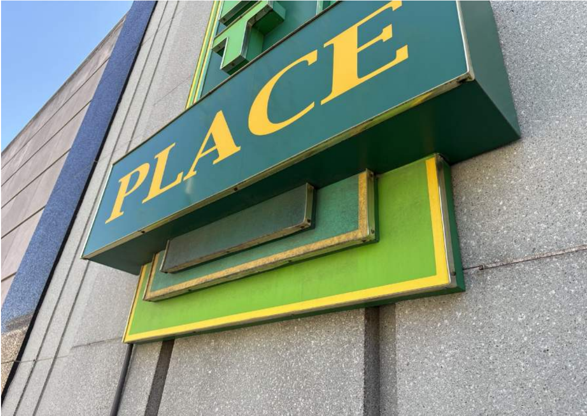
IMAGE 9: Exterior - looking south at close up view of existing signage wall-mounted to cut limestone cladding (photo from boom lift)
