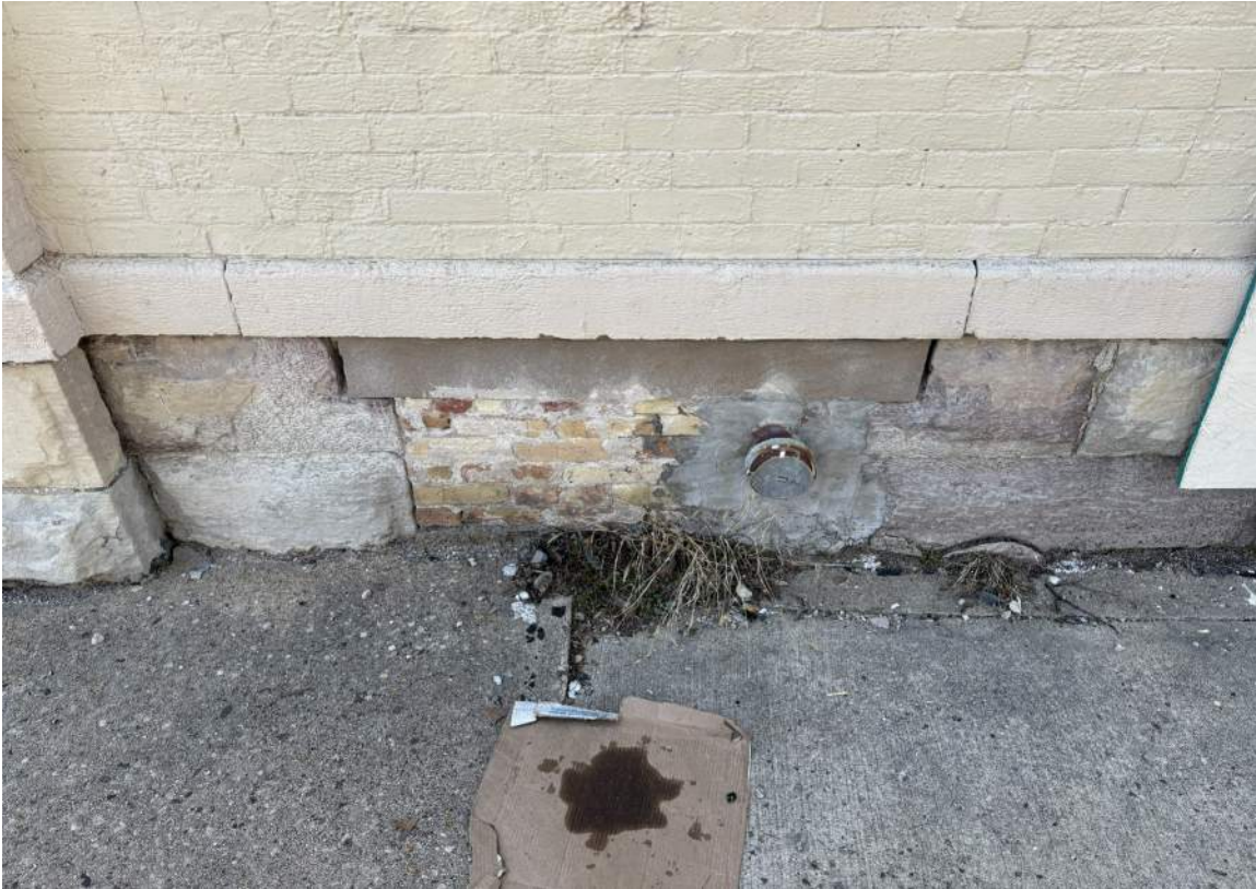
IMAGE 34: Exterior - looking down at existing brick infill at basement opening and existing replacement lintel
