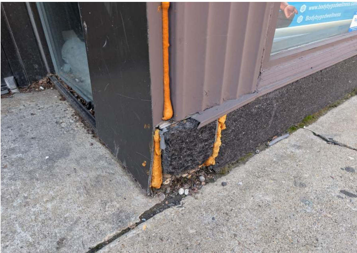
IMAGE 5: Exterior - looking down at deteriorated cast granite panels and existing spray foam insulation
