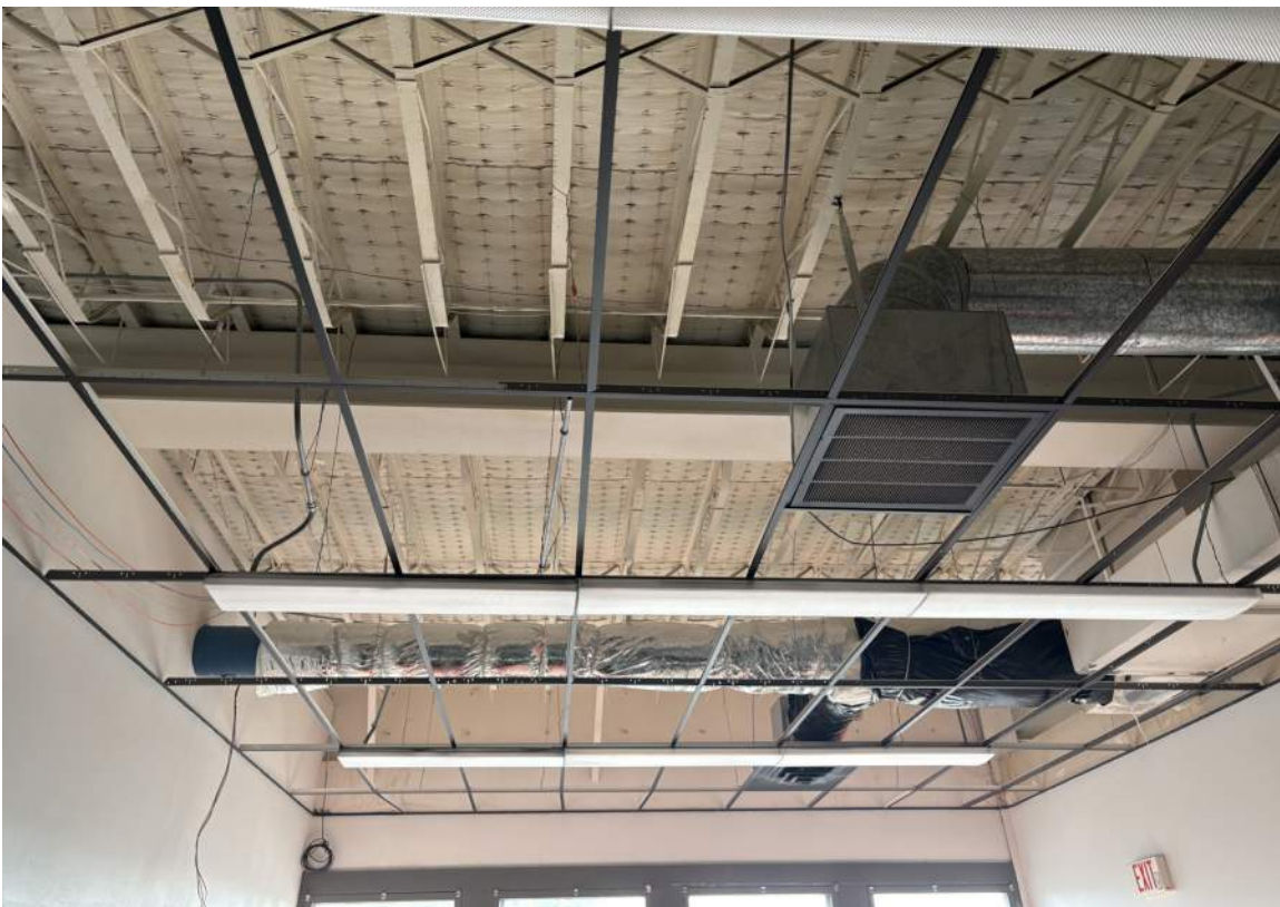
IMAGE 109: Level 02 - 1949 Structure - looking east and up at existing ACT ceiling grille in foreground and open steel roof joists beyond
