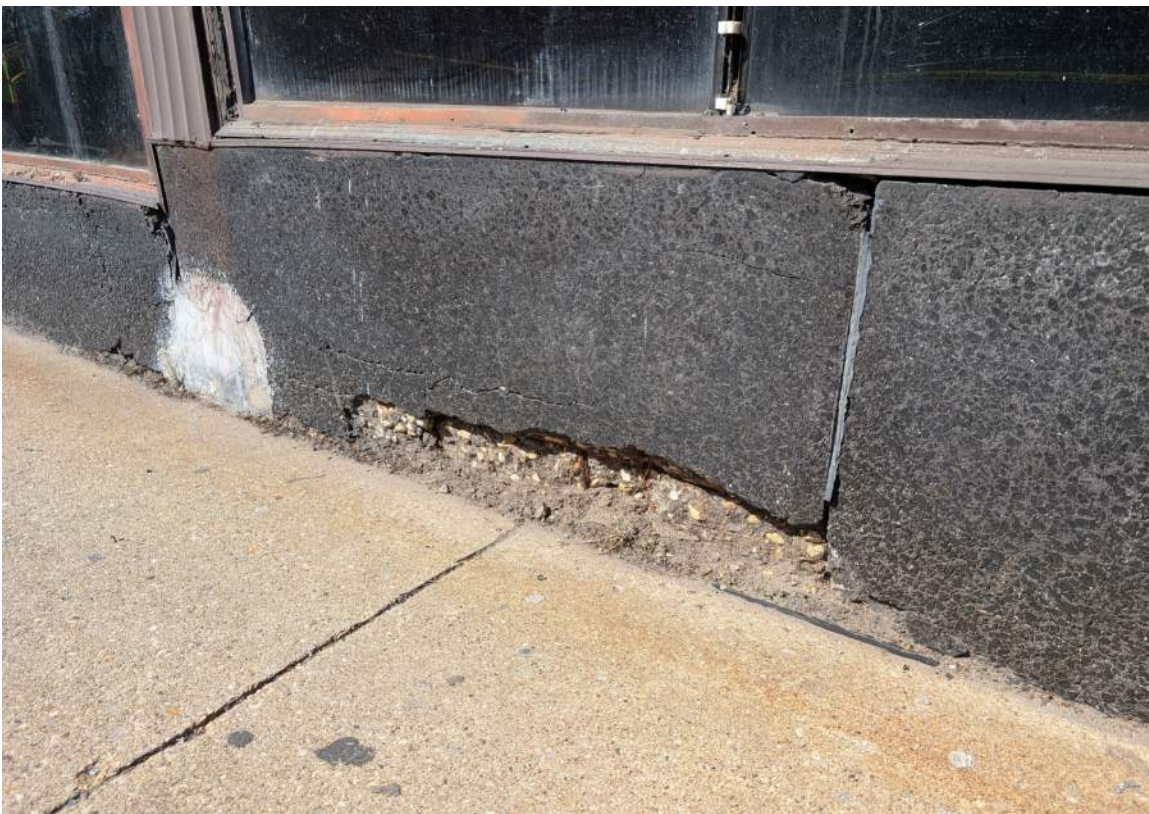
IMAGE 24: Exterior - looking down at broken and missing portion of cast granite panels; existing parking present on the left hand side of photo
