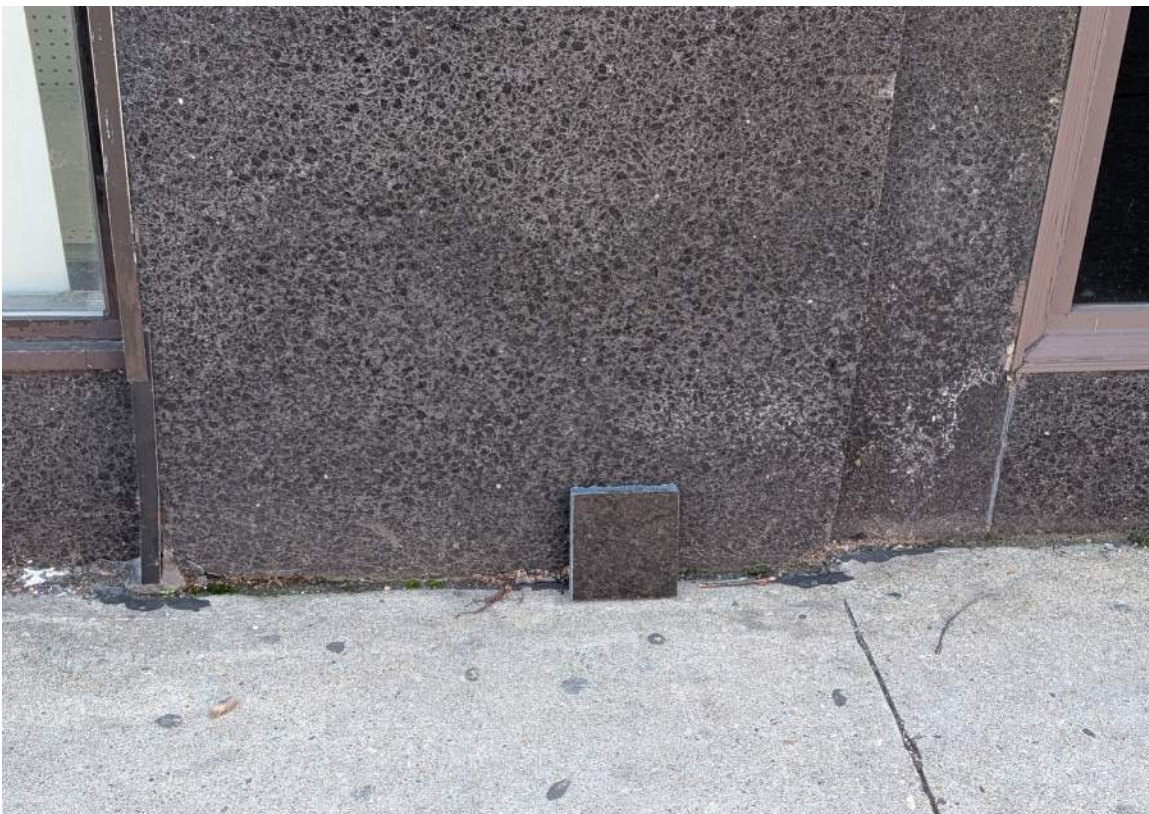
IMAGE 17: Exterior - looking down at existing cast granite panels at grade with sample of proposed replacement granite material in foreground (see attachments for additional info)
