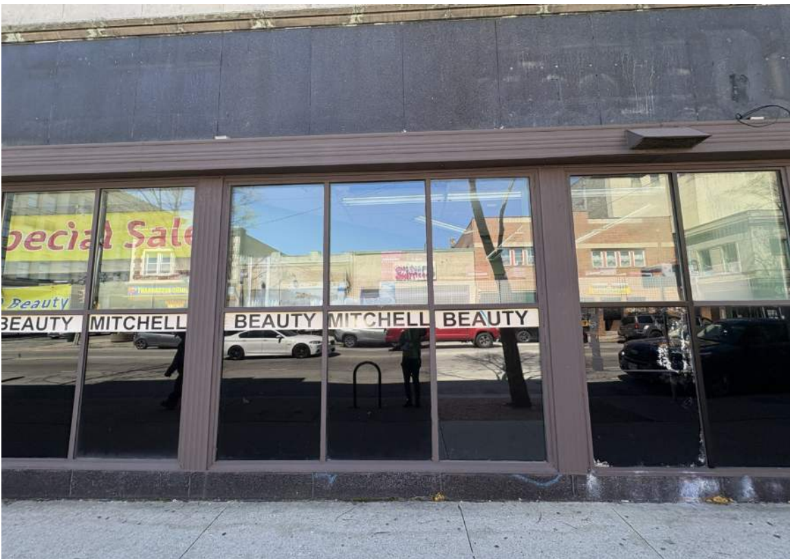
IMAGE 7: Exterior - looking south at existing storefront system and fluted bronze header and mullions
