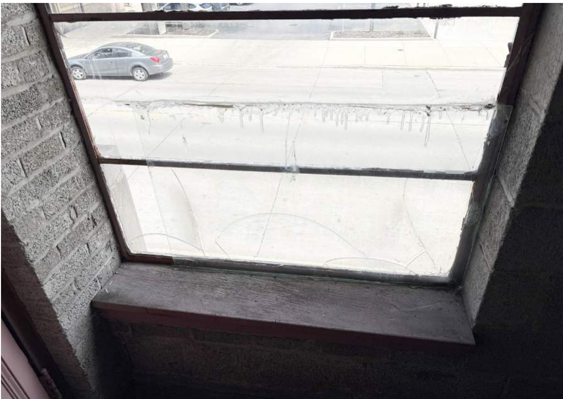
IMAGE 102: Mezzanine - 1949 Structure - inside staircase looking east at original steel sash window without interior storm window
