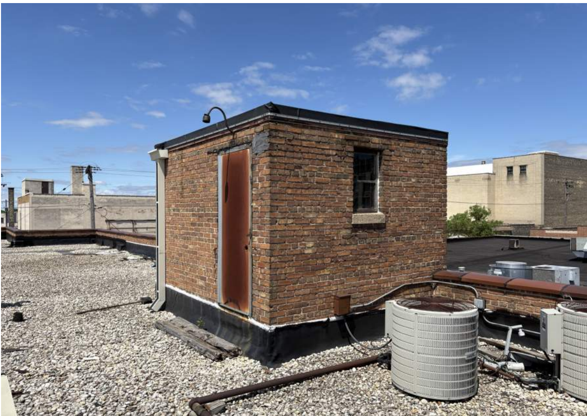
IMAGE 165: Rooftop - 1949 Structure - looking northwest at existing passenger elevator overrun
