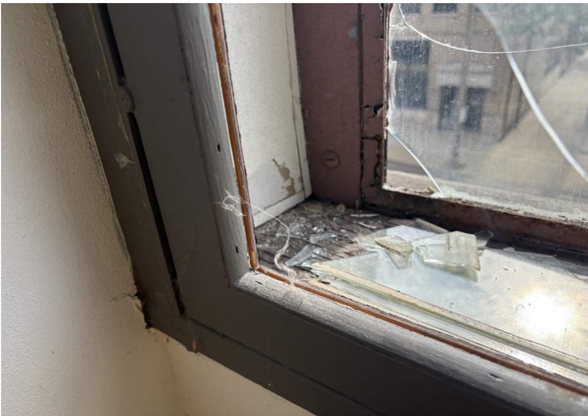
IMAGE 107: Level 02 - 1949 Structure - looking northeast at existing interior wood storm window in foreground and original steel sash window beyond
