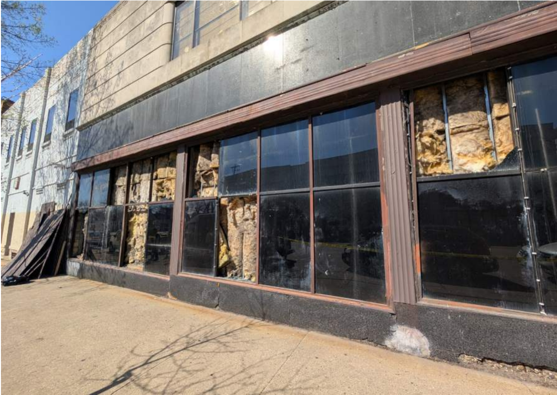
IMAGE 23: Exterior - looking southwest at existing storefront system - broken panes of glass and exposed insulation on backside of interior furring wall beyond
