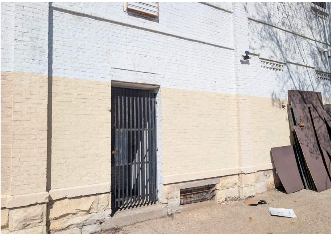
IMAGE 33: Exterior - looking northwest at existing opening which has been partially infilled at the head
