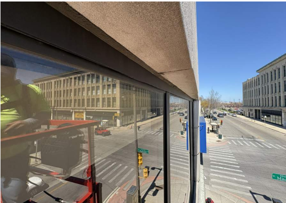
IMAGE 26: Exterior - looking north at underside of existing cut limestone window headers (photo from boom lift)
