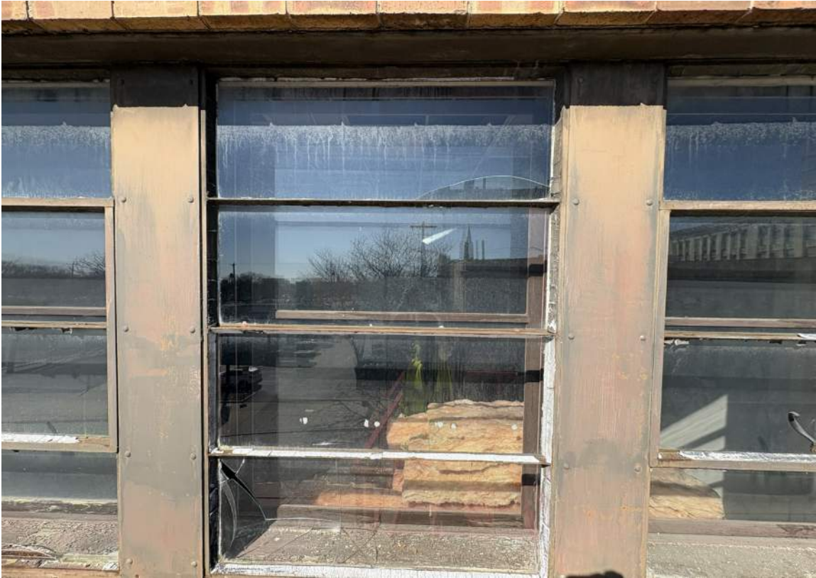
IMAGE 40: Exterior - looking west at original steel sash windows at level 02 (photo from boom lift)
