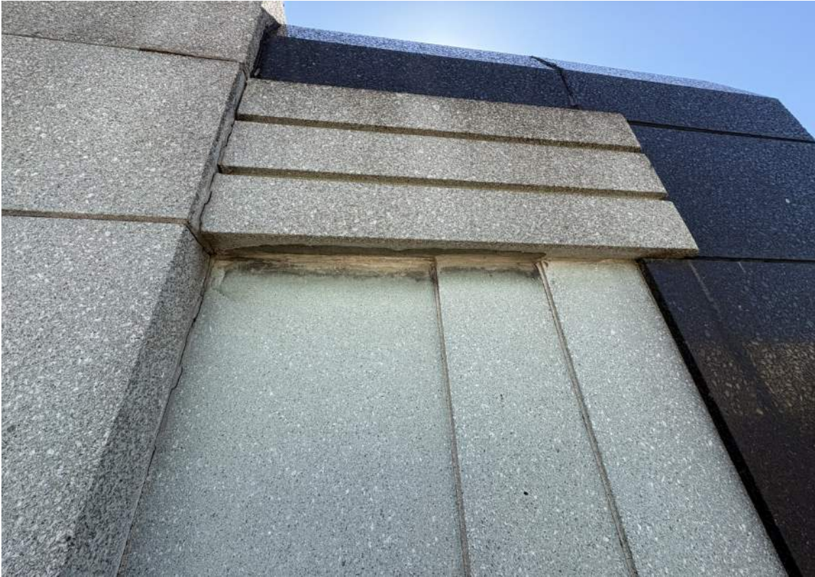
IMAGE 11: Exterior - looking up at existing cast granite and cut limestone - detailing where ornamentation steps up at roofline (photo from boom lift)
