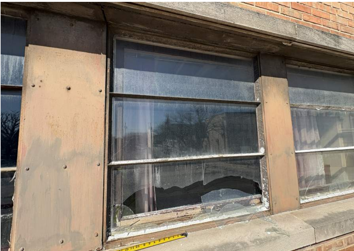
IMAGE 39: Exterior - looking west at original steel sash windows at mezzanine level (photo from boom lift)
