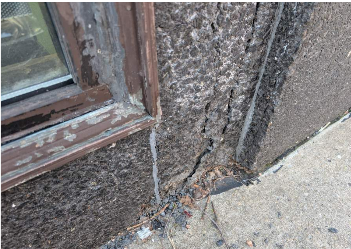
IMAGE 15: Exterior - looking down at deteriorated cast granite panels with existing fill at through cracks; base of existing storefront system with perimeter trims
