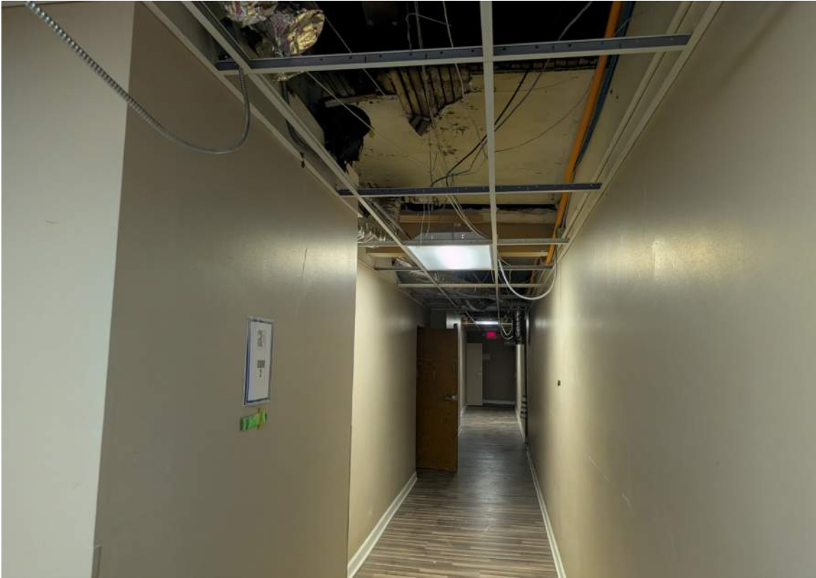
IMAGE 156: Level 02 - pre-1888 Structure - looking west down existing corridor - small remnant of plaster ceiling on wood lath overhead
