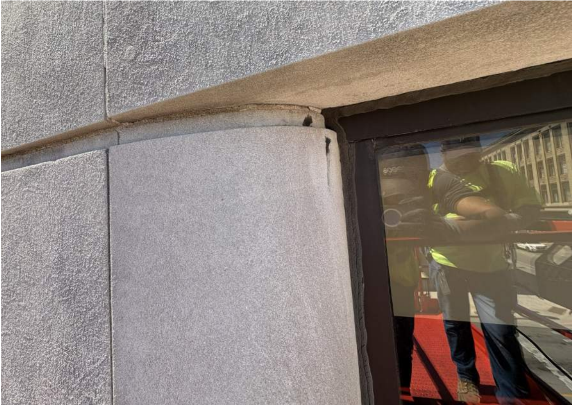
IMAGE 27: Exterior - looking up at existing storefront window and rounded portion of existing cut limestone at window jamb (photo from boom lift)
