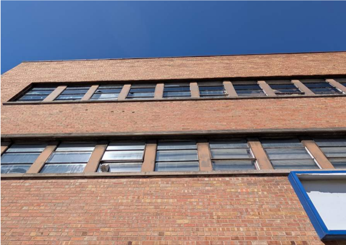
IMAGE 38: Exterior - looking up at original steel sash windows with limestone lintels and sills
