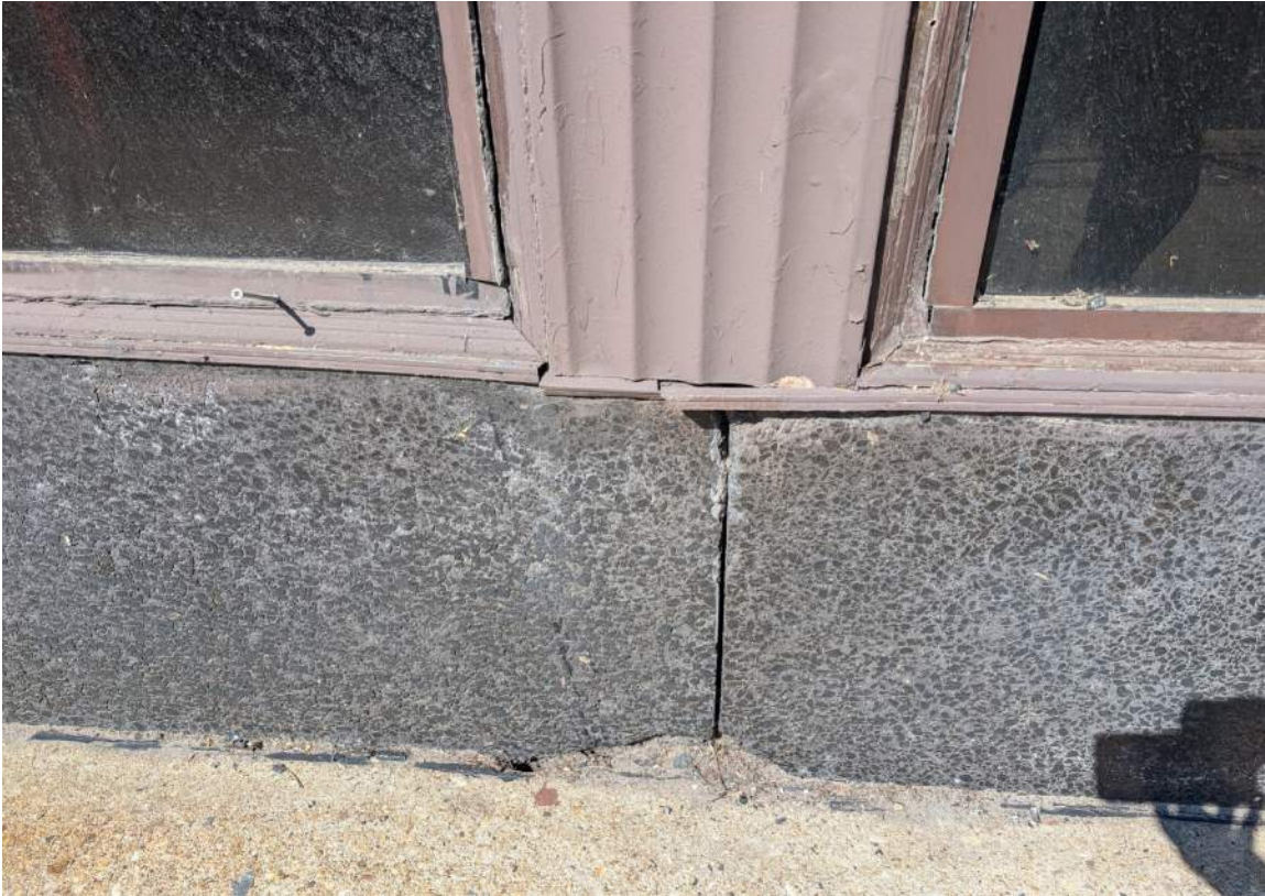
IMAGE 16: Exterior - looking down at existing cast granite at grade, painted, bronze fluted mullion, and existing storefront system with perimeter trims
