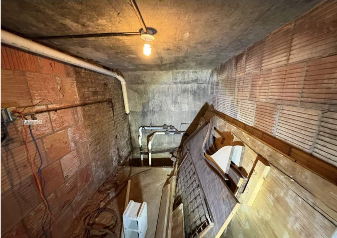
IMAGE 54: Basement - 1949 Structure - vault beneath sidewalk - looking east at existing exterior concrete vault wall and clay tile side walls
