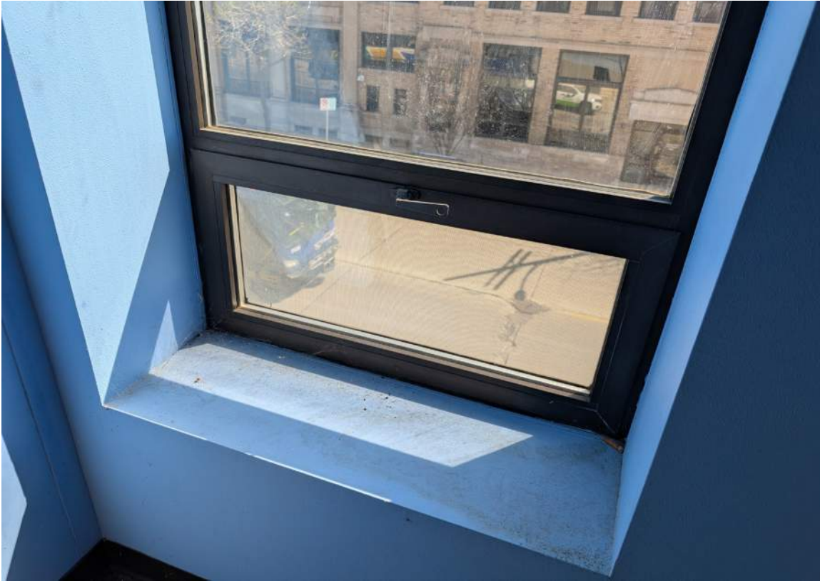
IMAGE 140: Level 02 - 1911 Structure - looking east at existing storefront window with lower operable hopper
