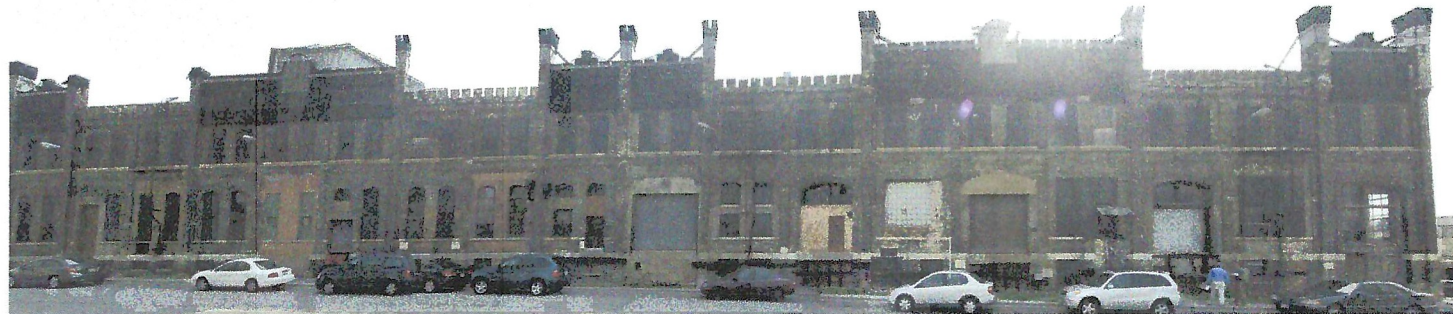
3 CURRENT CONDITION PHOTOGRAPH - FOR REFERENCE ONLY
