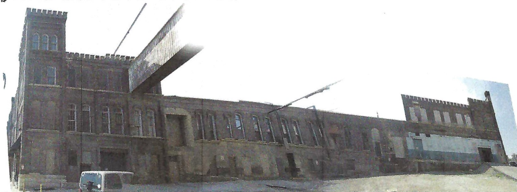
3 CURRENT CONDITION PHOTOGRAPH - FOR REFERENCE ONLY
