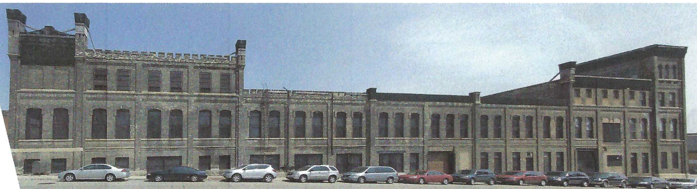
3 CURRENT CONDITION PHOTOGRAPH - FOR REFERENCE ONLY
