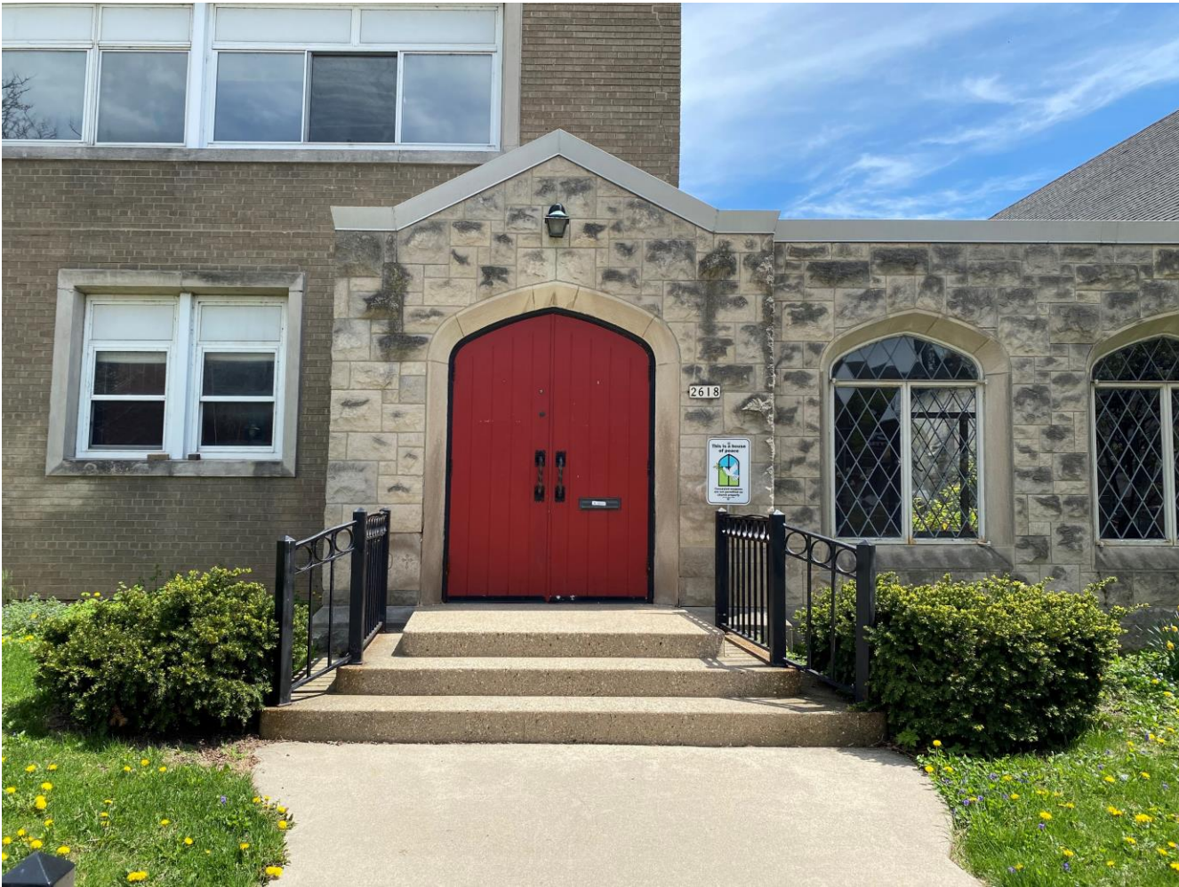
Existing limestone conditions with extensive charcoal color patina
