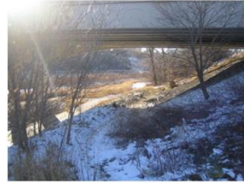
VIEW SOUTH TO EXISTING BIKE PATH
