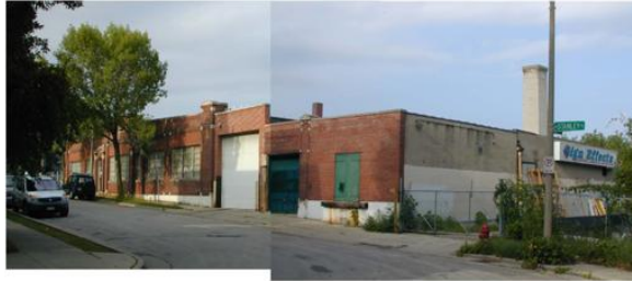
WEST FACADE, 2362 N. STANLEY
