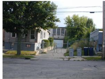
NORTH ALLEY ACCESS TO 2362 N. STANLEY
