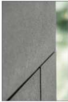
04 FCMT-01 MATERIAL: FIBER CEMENT WALL PANELS COLOR: CLP-02 TYPE: AS SHOWN FINISH: VERTICALLY CORRUGATED "HART LOOM" FINISH LOCATION: 2ND AND THIRD FTH FLOORS
