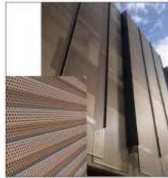
07 PERF-01 MATERIAL: PERFORATED CORRUGATED METAL PANELS COLOR: CLP-02 FINISH: TB0 FINISH LOCATION: 2ND AND THIRD FTH FLOORS
