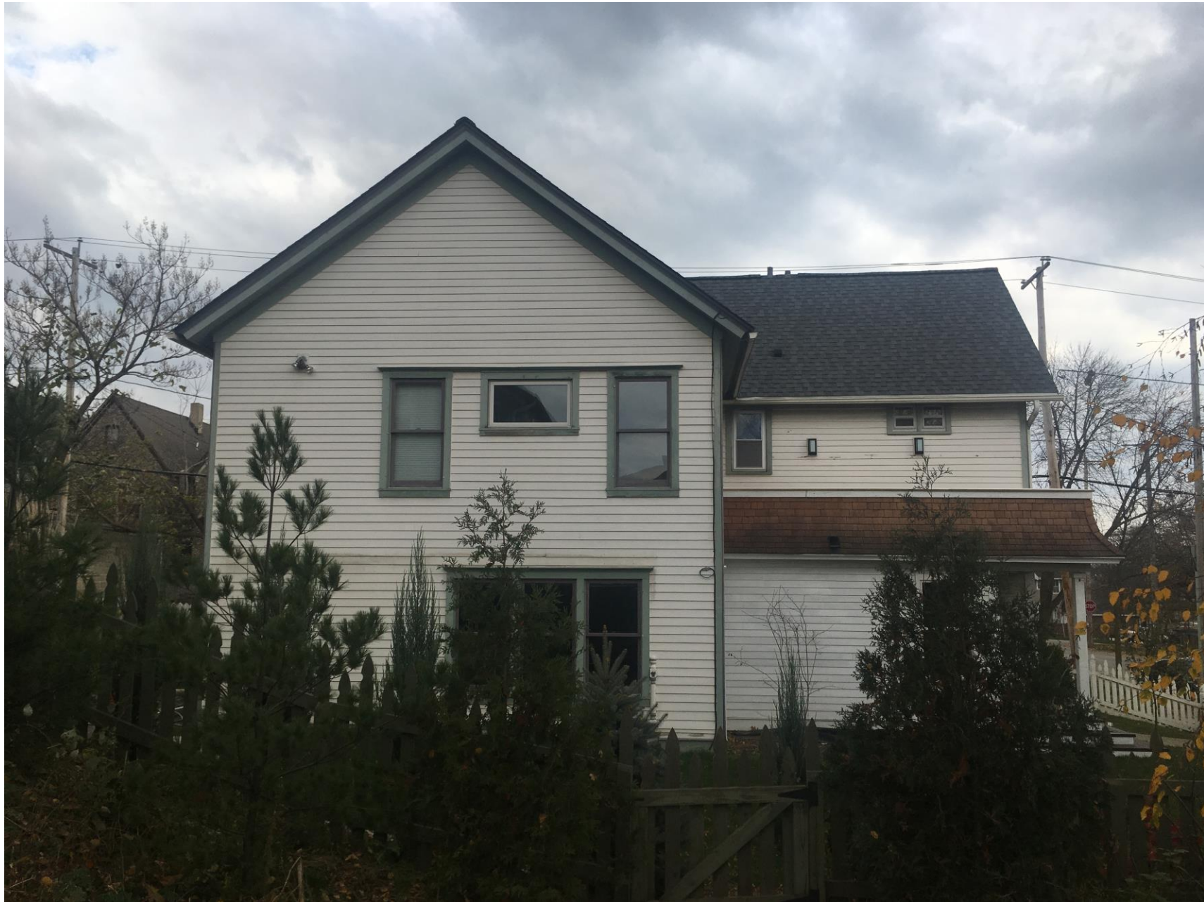
Existing conditions west elevation
