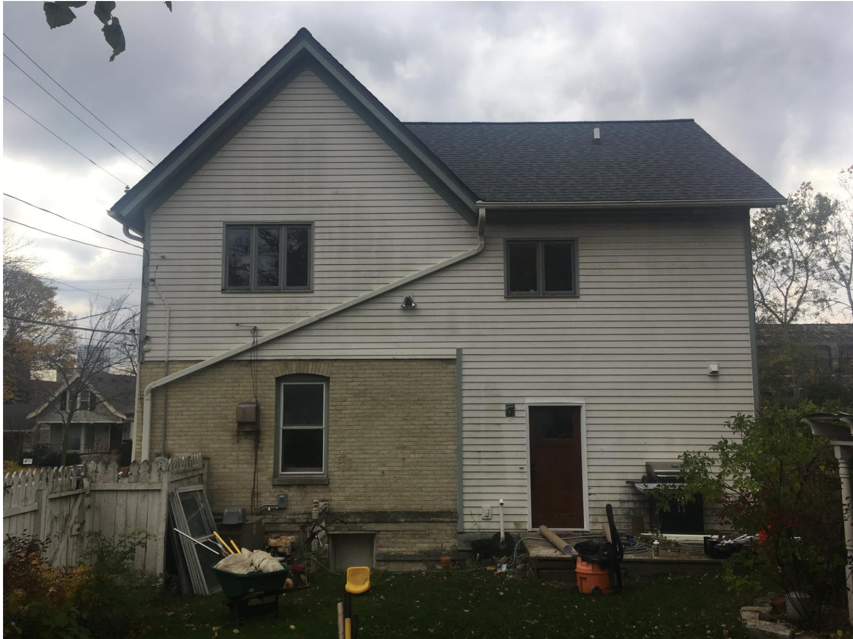
Existing conditions, north elevation
