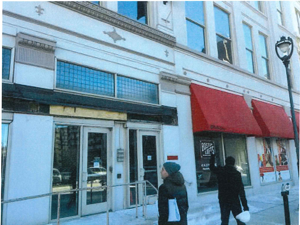
4TH ST. OFFICE ENTRY (EXISTING CANOPY REMOVED) - LOOKING SOUTH
