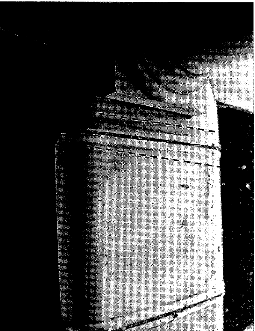
Figure F: Open joints between railing units allow water to seep into railings and walls, hastening the deterioration of terra cotta and masonry below.
