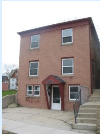
3710 W Lisbon – Rental Rehab
