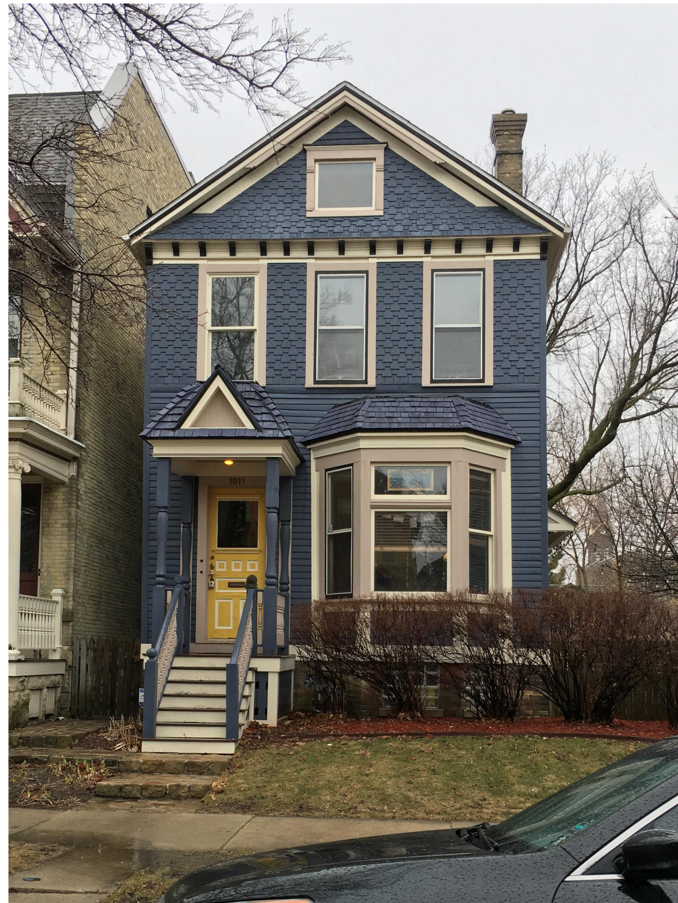
1 EXISTING EAST ELEVATION - NO CHANGE TO THIS ELEVATION SCALE: NOT TO SCALE
