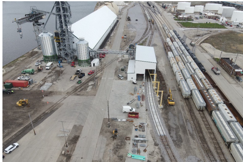
Figure 5: Phase 1 Progress – April 2023
