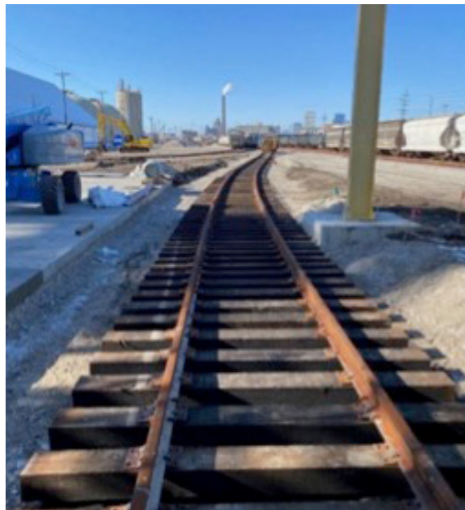
Figure 12: New Rail Provided by the Port
