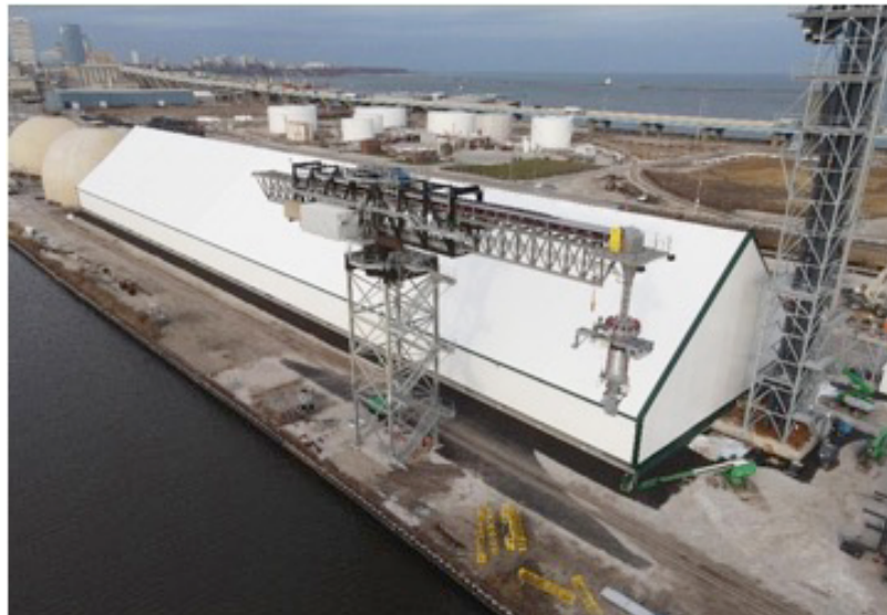
Figure 7: DDG Flat Storage Building and Ship Loader
