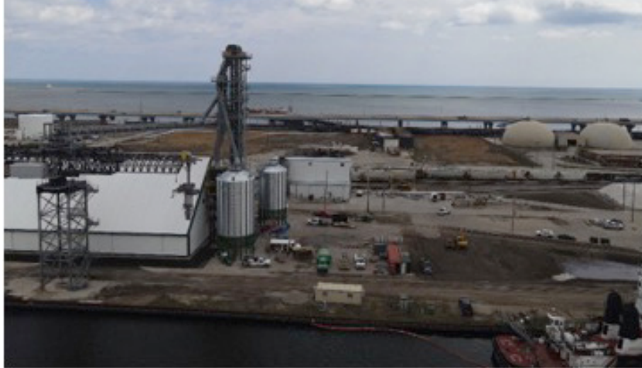
Figure 4: Phase 1 Progress – April 2022
