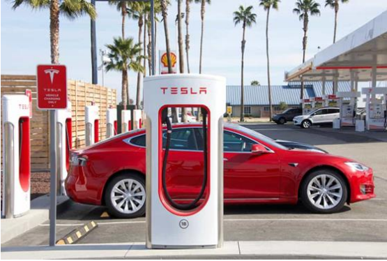
Figure 1 - Tesla Fast Charging Station
