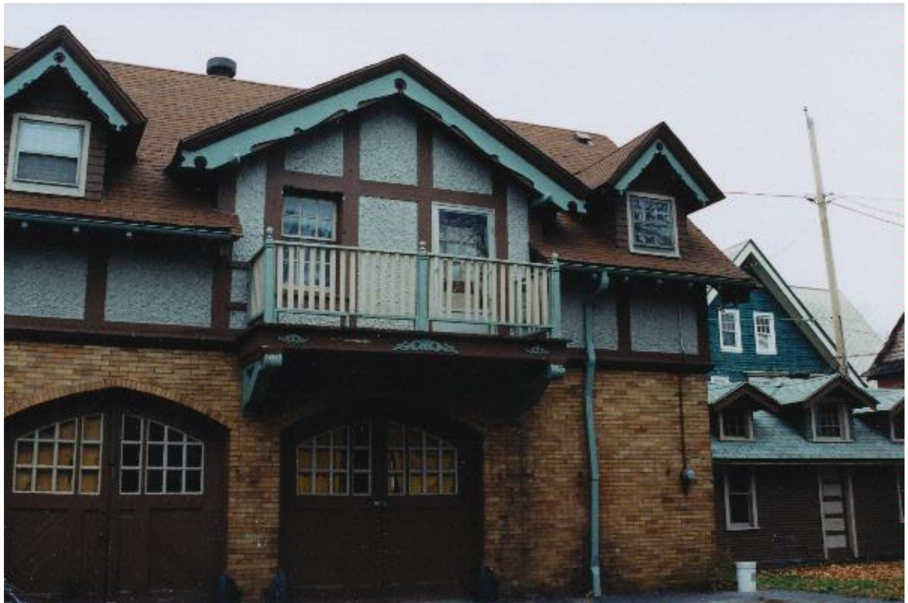
Coach house at 3014 W. McKinley Boulevard
