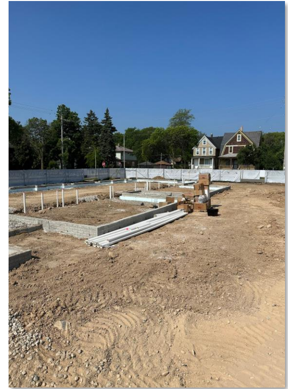
Townhouses are backfilled and underground plumbing
