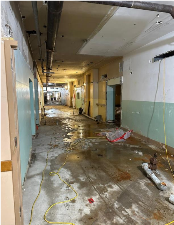
Demolition to create new corridor
