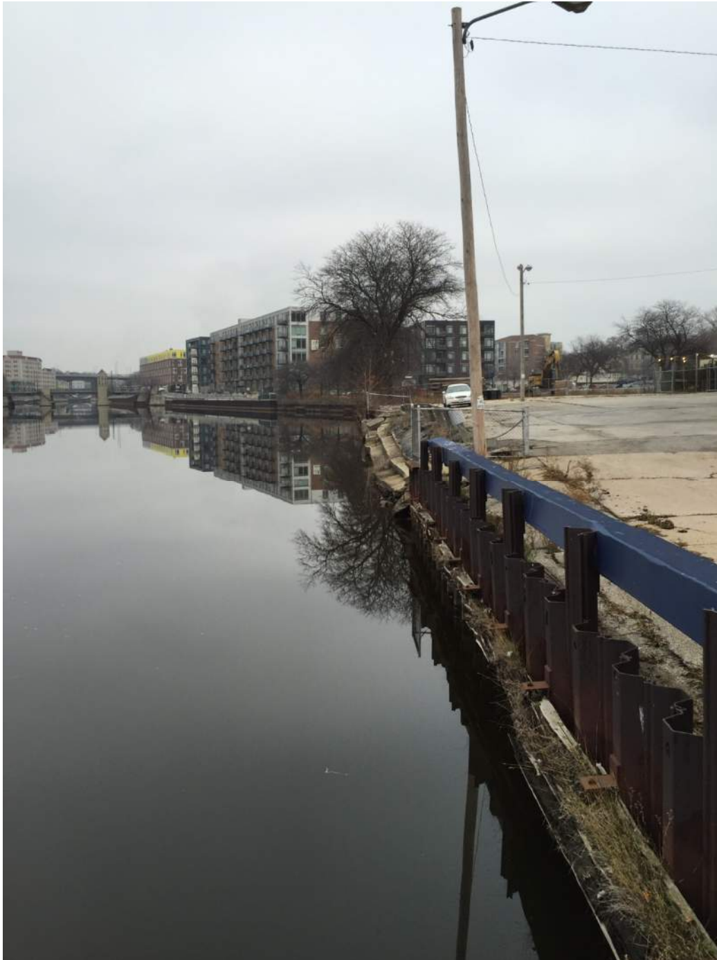
Seawall looking north
