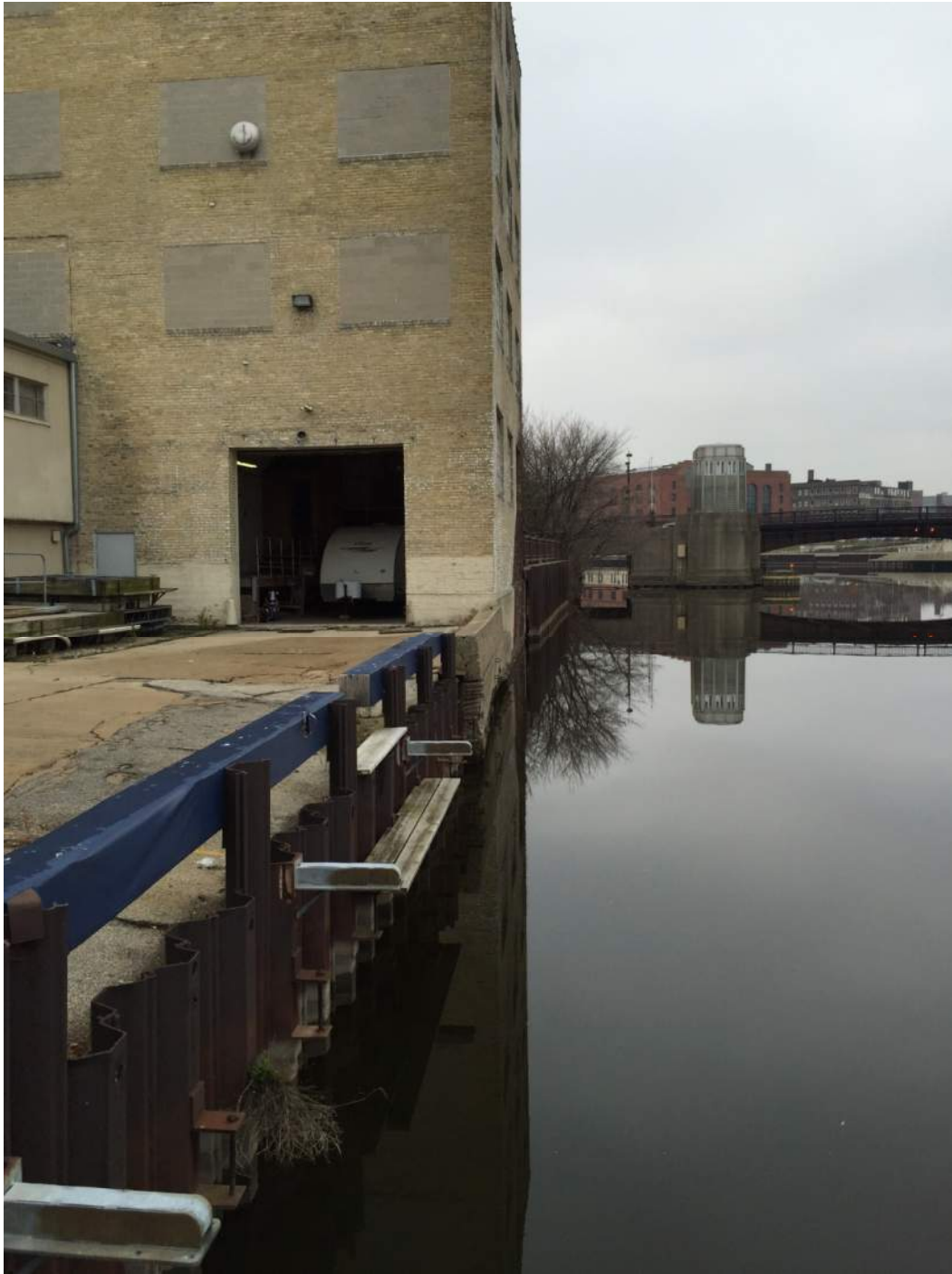
Seawall looking south
