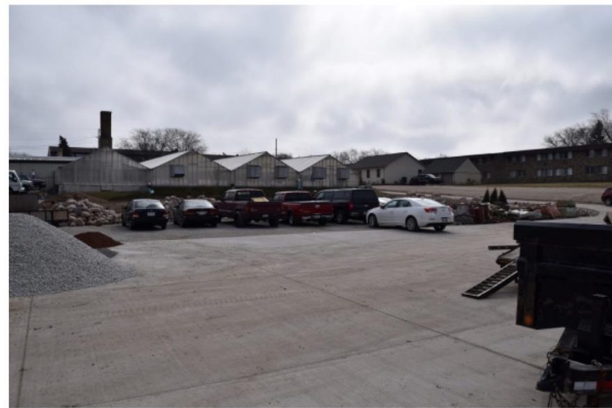
BUILDINGS 2 & 3 – looking east from center of property
