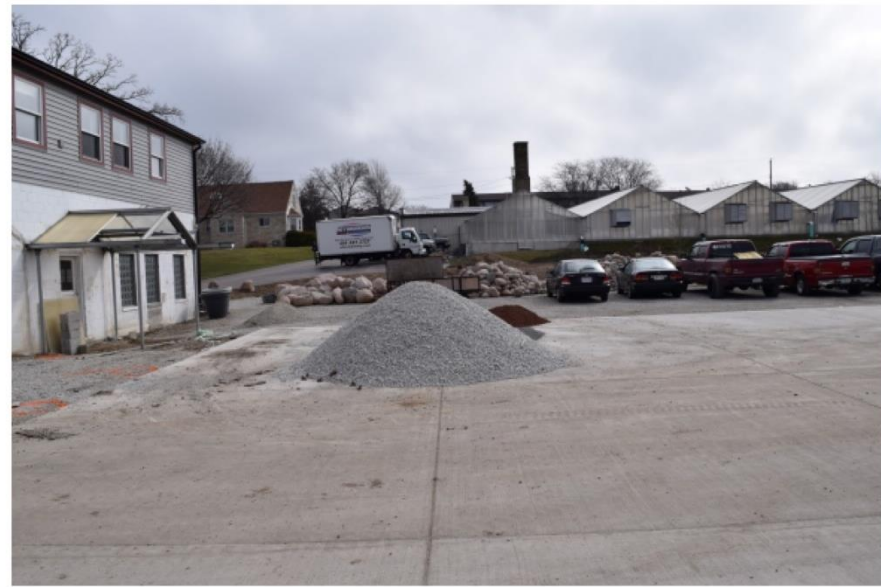
BUILDINGS 5, 1, 2, & 3 – looking east from center of property
