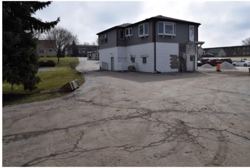
BUILDINGS 1 & 5 – looking east from center of north property line
