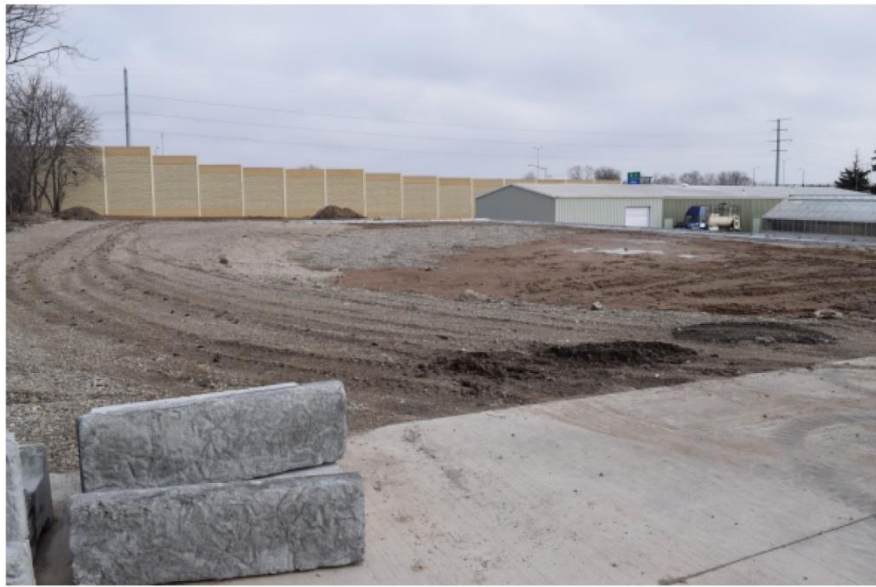
BUILDINGS 4 (future), 6, & 7 – looking north from southwest corner of property
