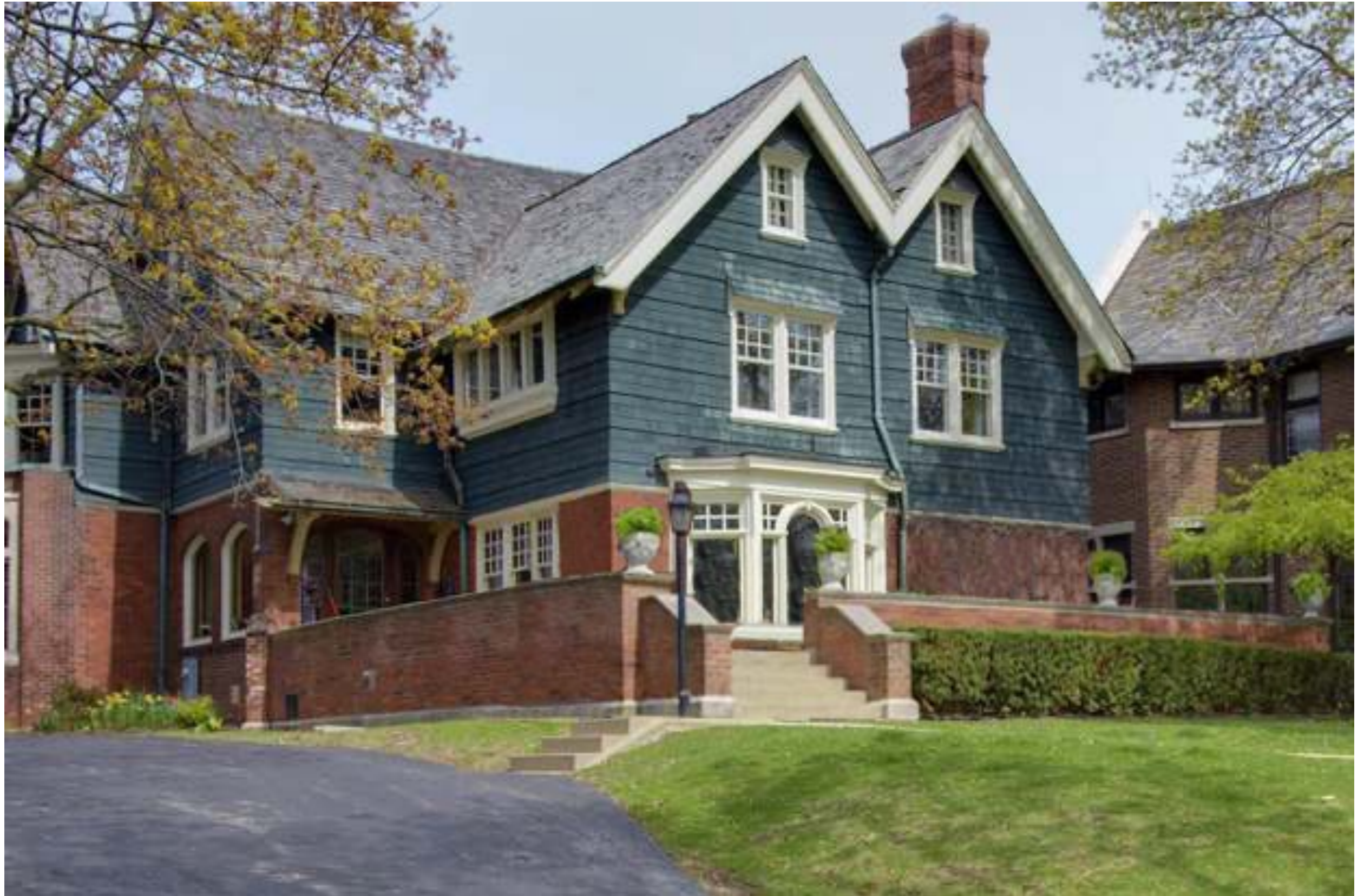
2239 N Terrace Ave - Deck Replacement - COA Application Nov 7, 2023
