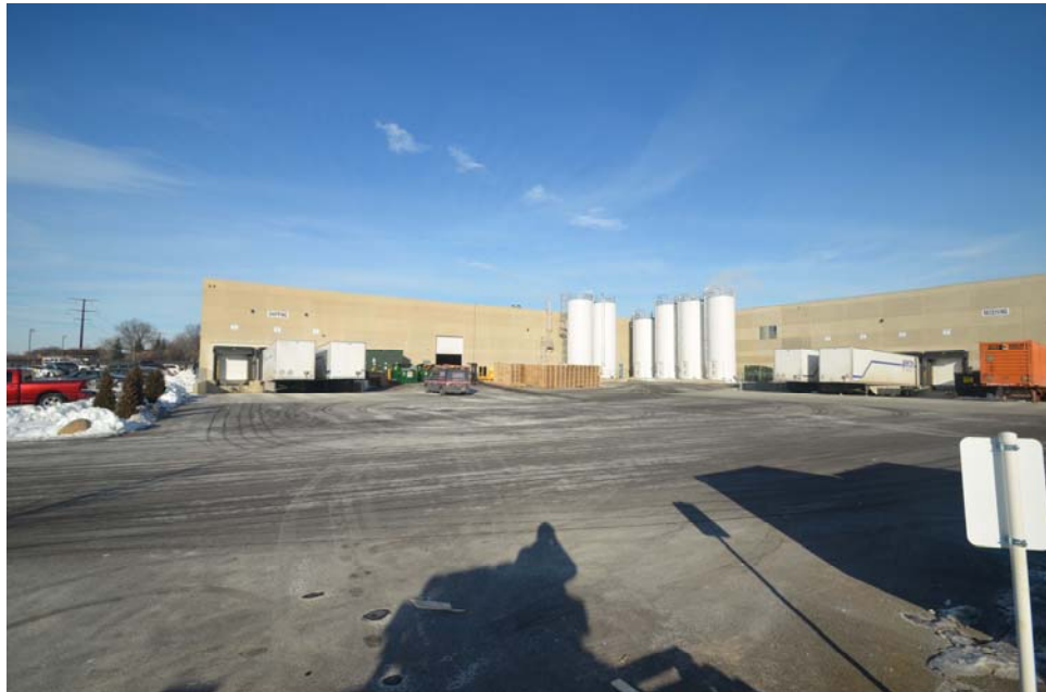
Looking Northeast – View of south façade of existing 2000 facility (2014 addition at right side of photo).
