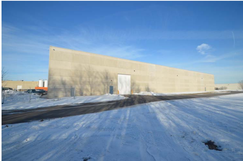
Looking North – View of south façade of existing 2014 addition (2000 facility beyond at left side of photo).
