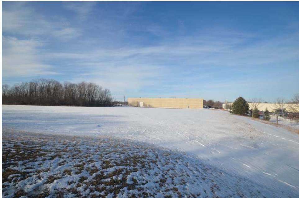
Looking North – View of proposed location of future addition (south façade of existing 2014 addition beyond).
