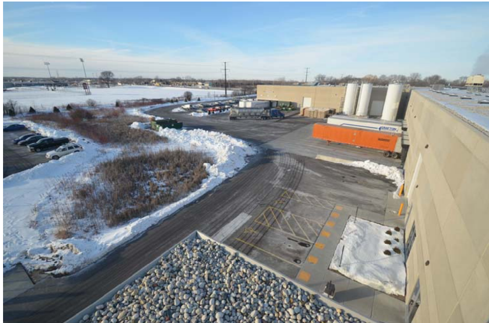
Looking Northwest from Roof of existing 2014 addition – View of 2000 facility, shipping docks and wetland.
