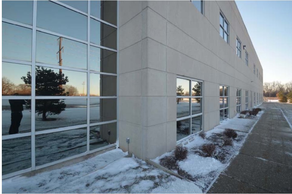
Exterior Material detail – West Façade of existing 2000 facility.
