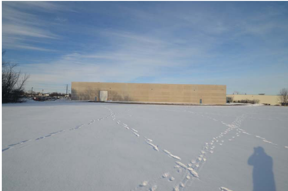
Looking North – View of south façade of existing 2014 addition from location of proposed addition.
