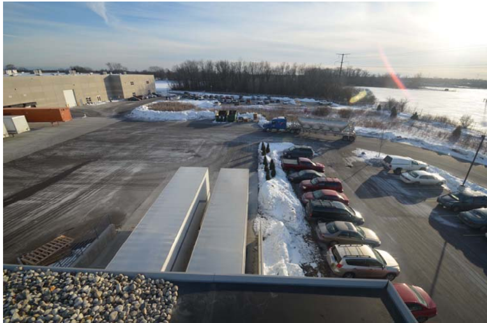
Looking South from Roof of existing 2000 facility – View of entry drive and shipping docks.
