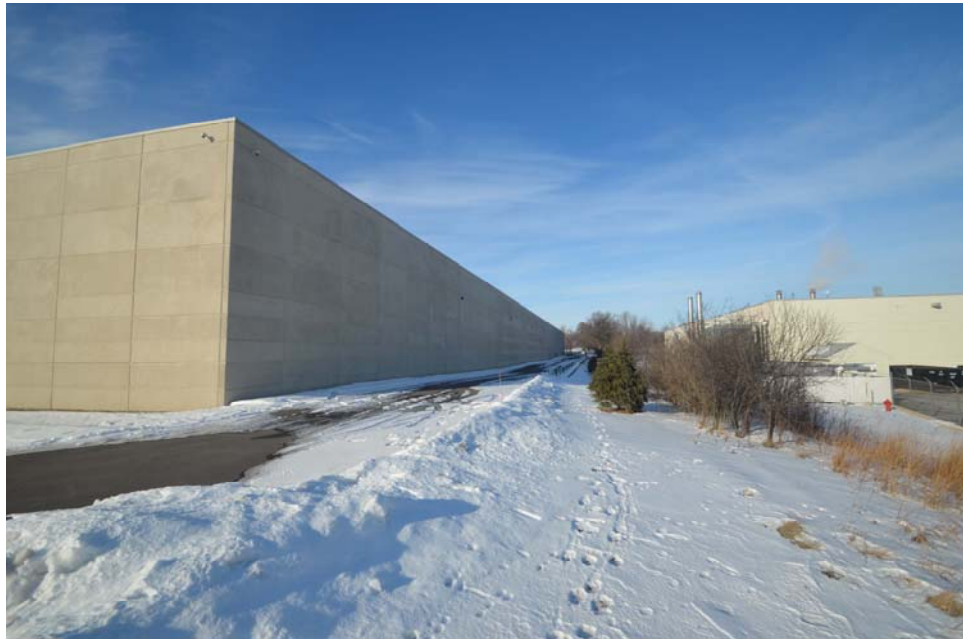
Looking North – View of east façade of existing 2014 addition along east property boundary.
