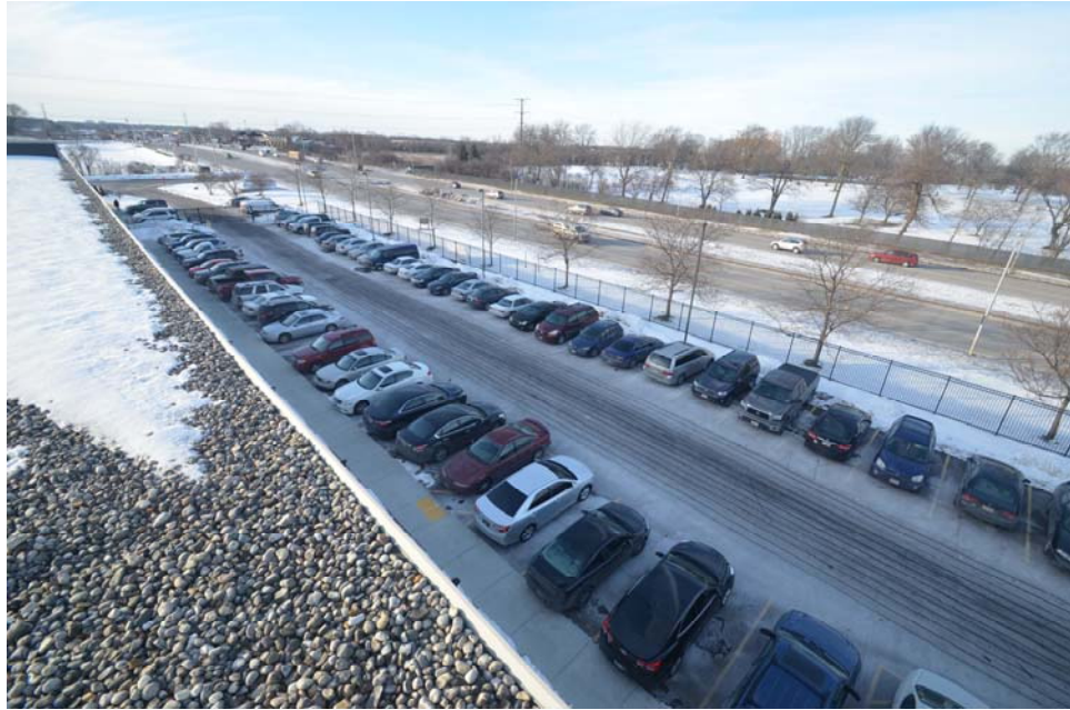
Looking Northwest from Roof of existing 2000 facility – View of north parking lot.
