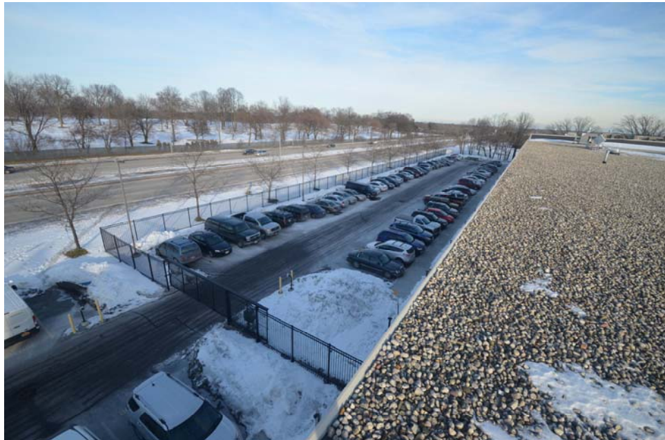
Looking Northeast from Roof of existing 2000 facility – View of north parking lot.
