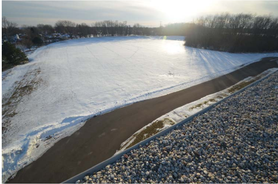
Looking Southwest from Roof of existing 2014 addition – View of fire apparatus access drive and proposed location of future addition.
