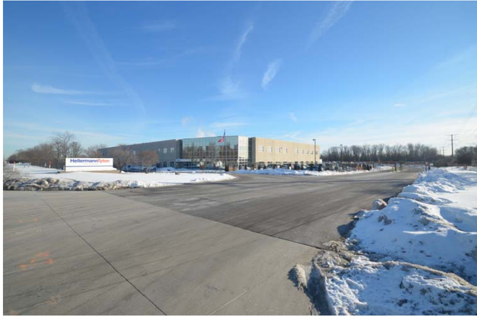
Looking Southeast – View of north and west façades of existing 2000 facility.
