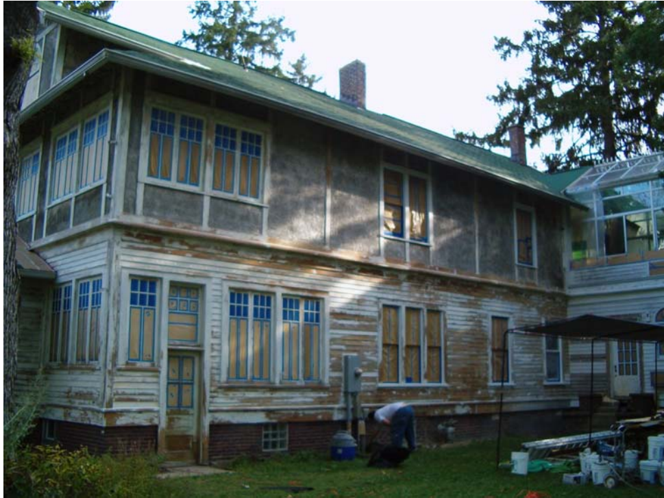
House in Clermont – with RS primer – applied 2003
