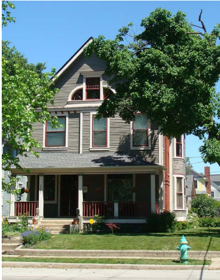
Front/West elevation – 2001 N Delaware
