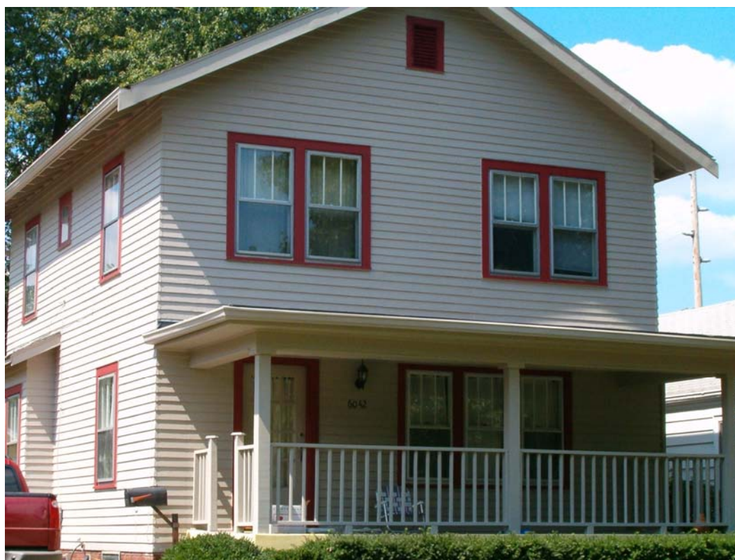
House in Broad Ripple (6042 Kingsley) – with RS primer and finish coat – finished 2003
