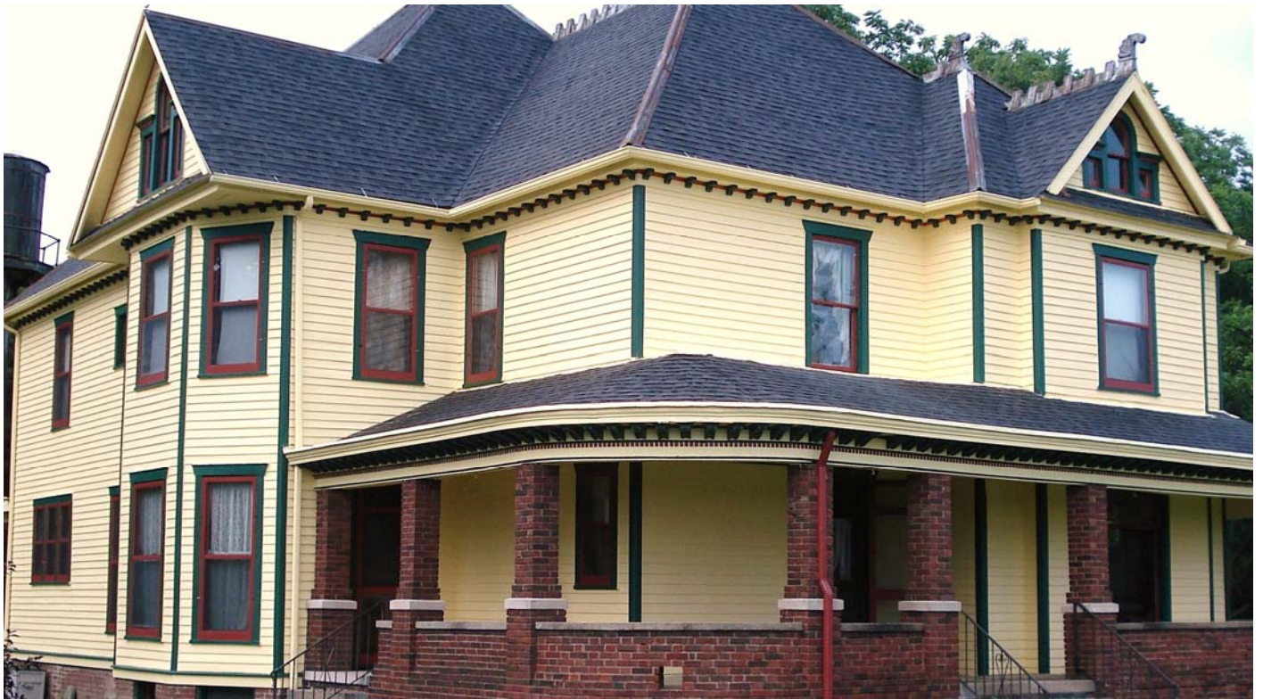
House in Crawfordsville – with RS primer and finish coat
