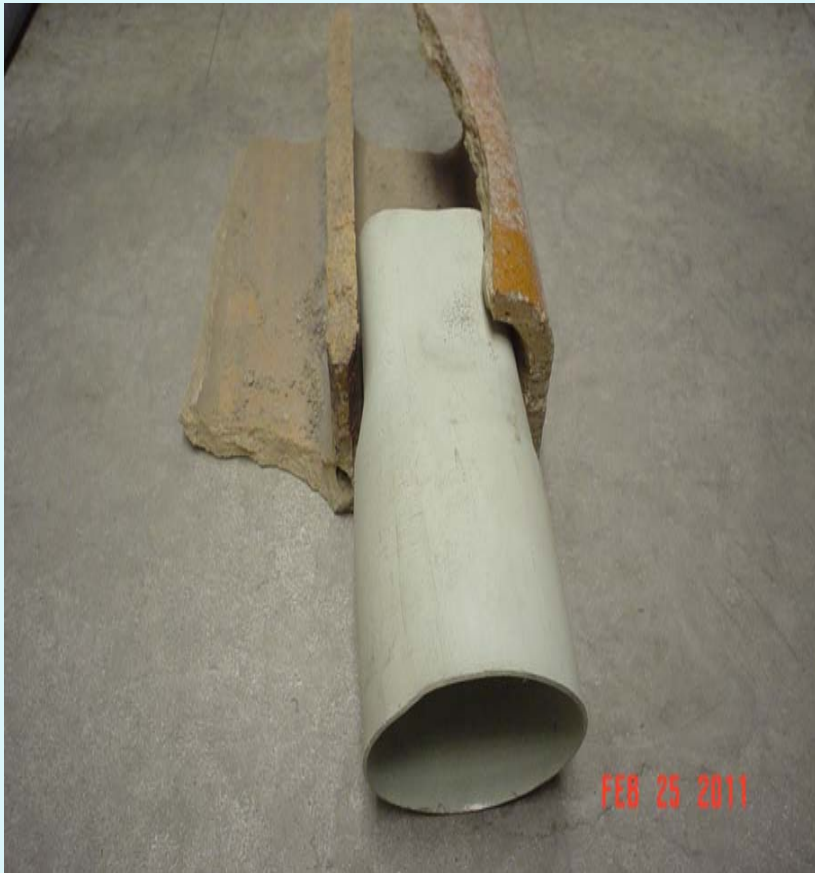
PVC Pipe in Clay Duct
