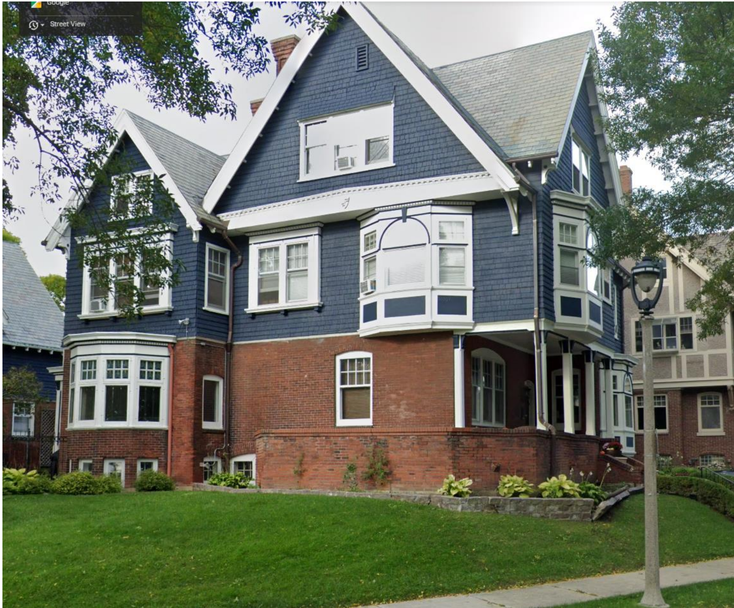
Present retaining viewed from south showing failed section at right of image.
