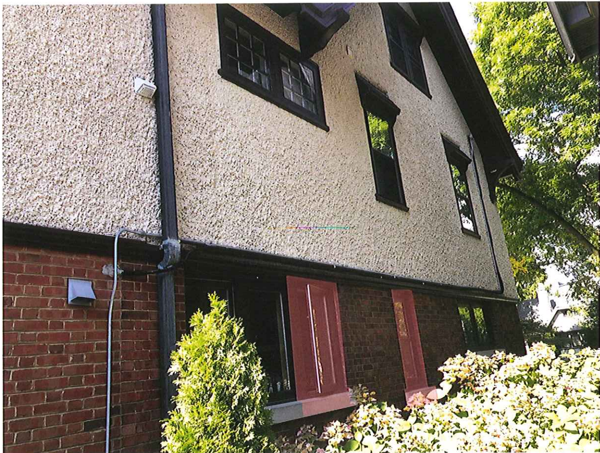
North Elevation from side yard
