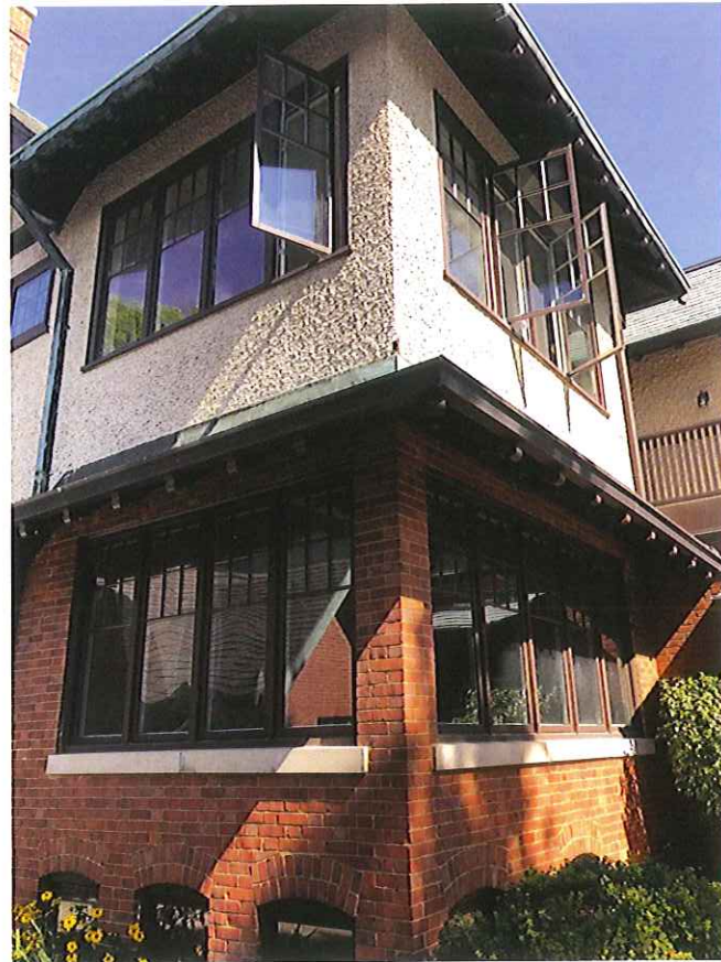
South East Corner
