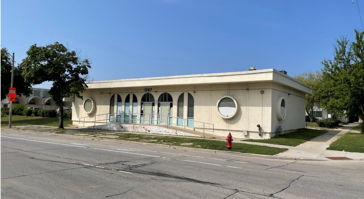
N. 6 th Street façade
