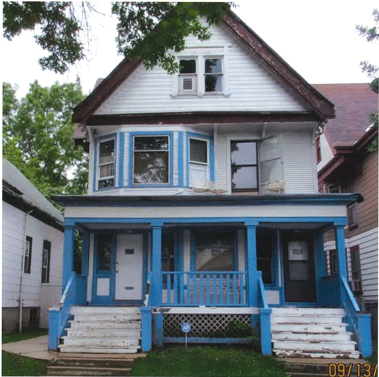
921-23 West Clarke Street
