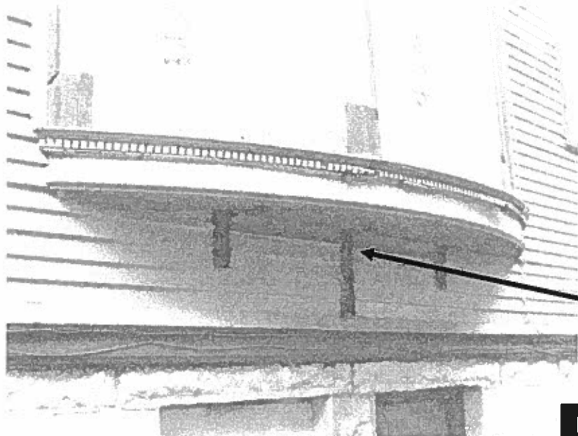
15. Missing soffit and fascia on southeast corner of east side gable.
