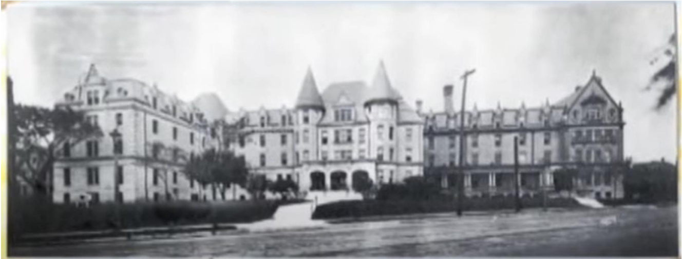
Figure 5: A ca. 1926 Photograph showing the 1926 section and changes made to the building by Fitzhugh Scott and MacDonald Mayer.
