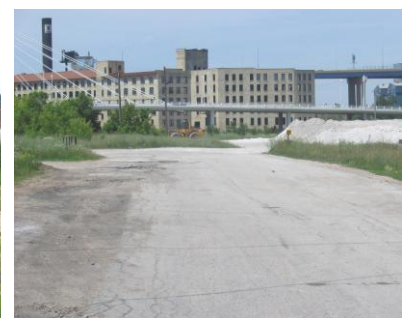
View looking west from 3 rd St.
