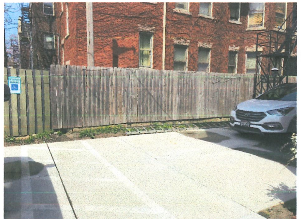
Wall is on the west side of the Mansion.
