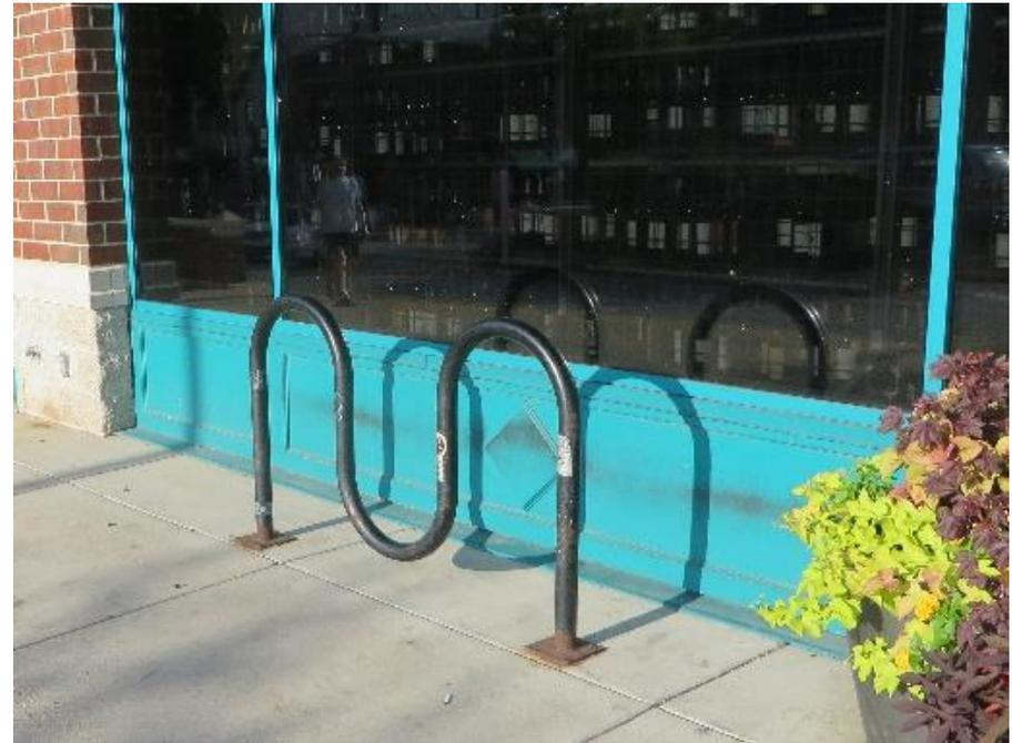
A discourage “wave” rack, it is mounted too close to wall to allow a bike to positioned in the intended perpendicular manner!
