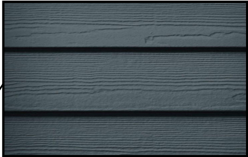
New Wood Siding Finish: Board size and color to match existing building.
