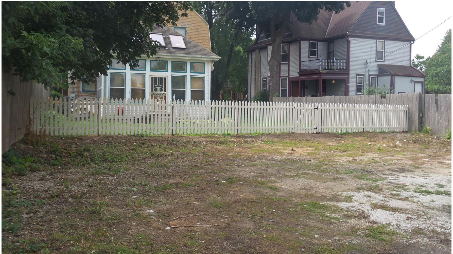
Photo of fence as installed.
