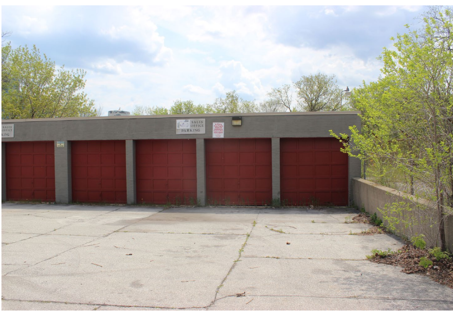
Block A existing structure
