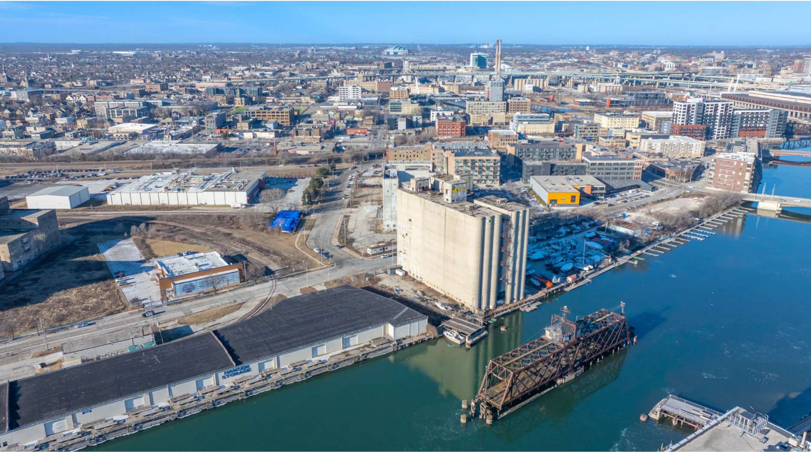
EXISTING SITE VIEW 6
