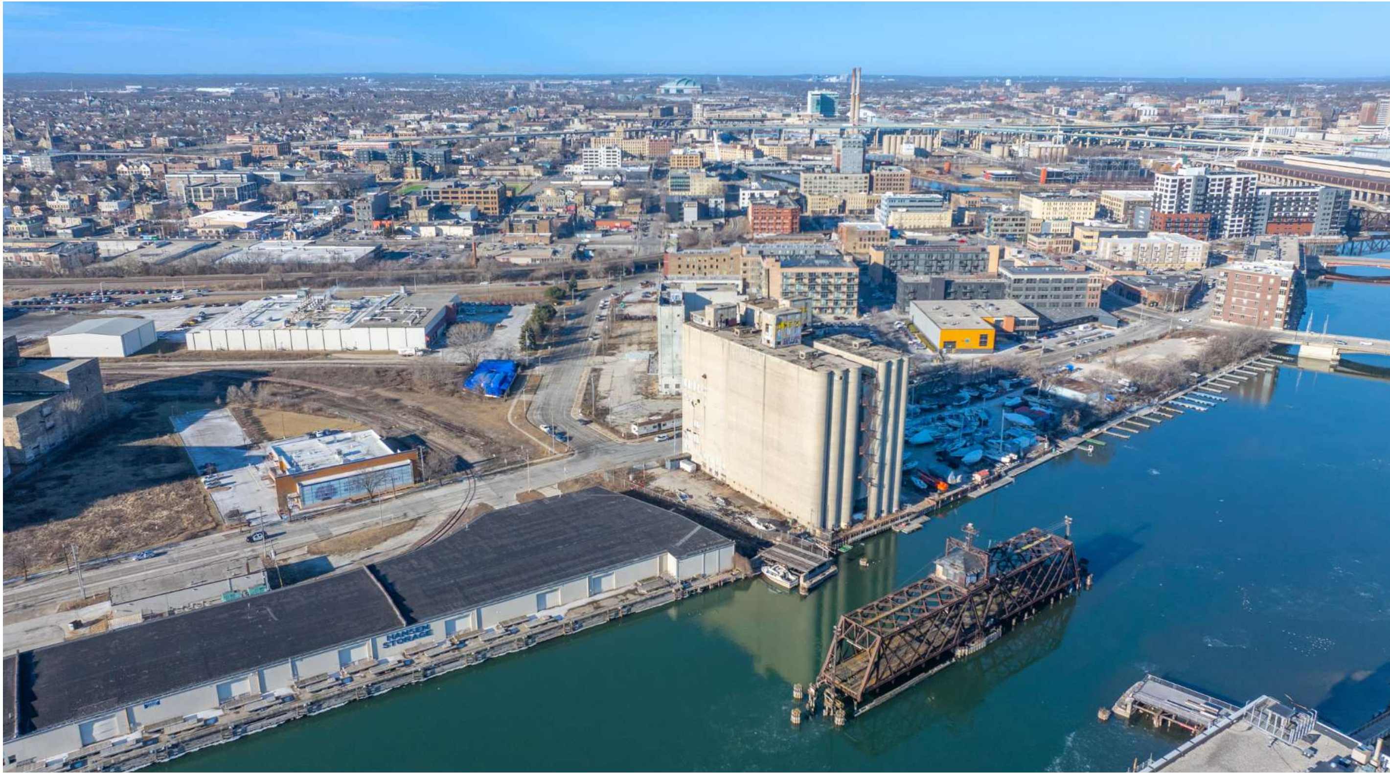
EXISTING SITE VIEW 6
