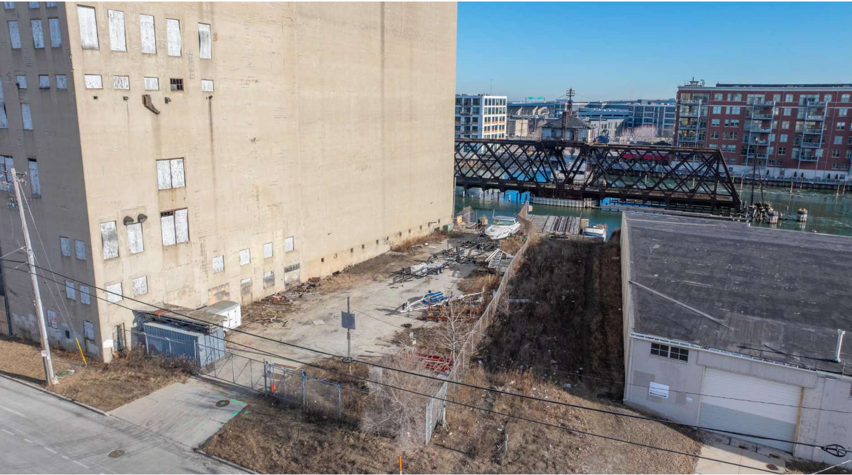
EXISTING SITE VIEW 1
