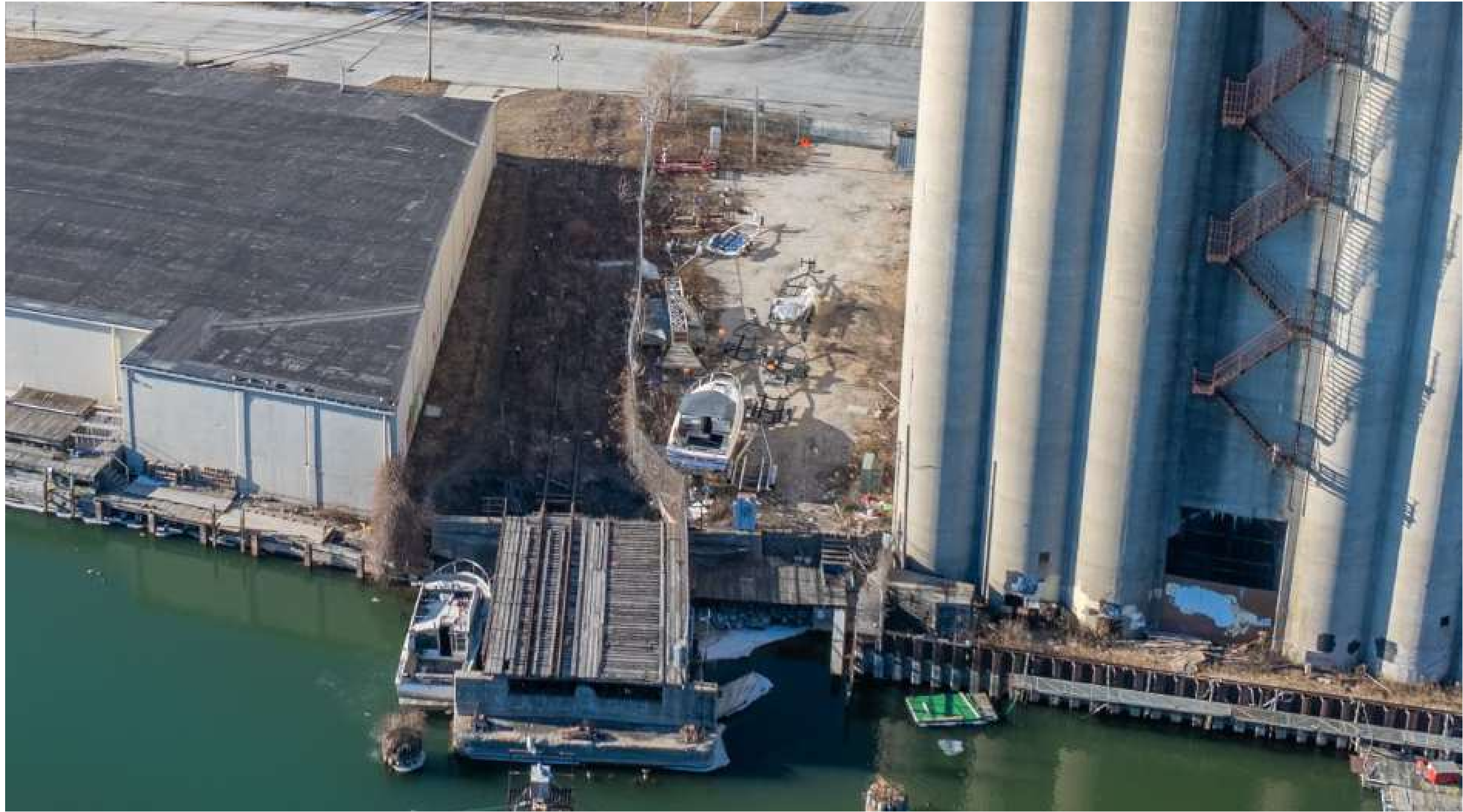
EXISTING SITE VIEW 4
