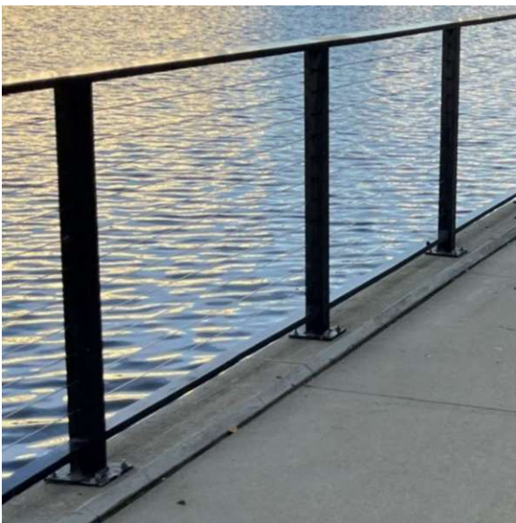
RIVERWALK RAILING - METAL CAP AND POST WITH CABLE RAIL
