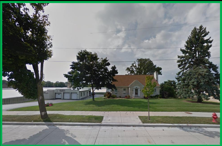
View from South 20 th Street, looking west
