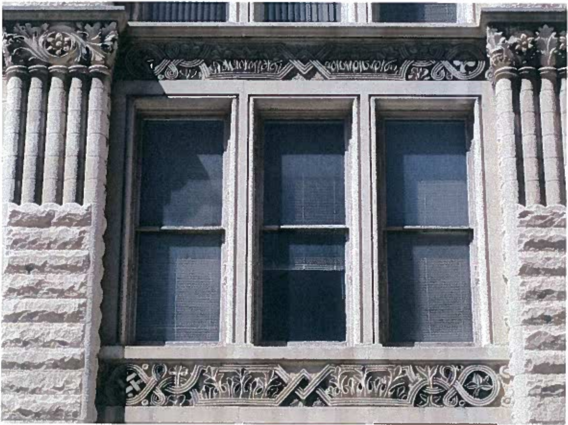
Photo 15: Third Floor window detail
