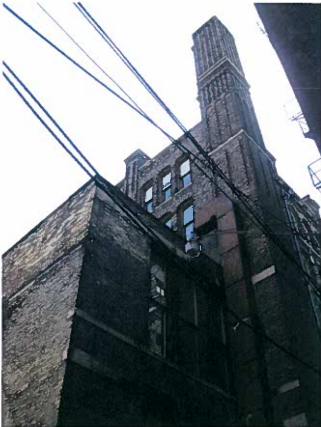
Photo 10: Alley Façade, looking South
