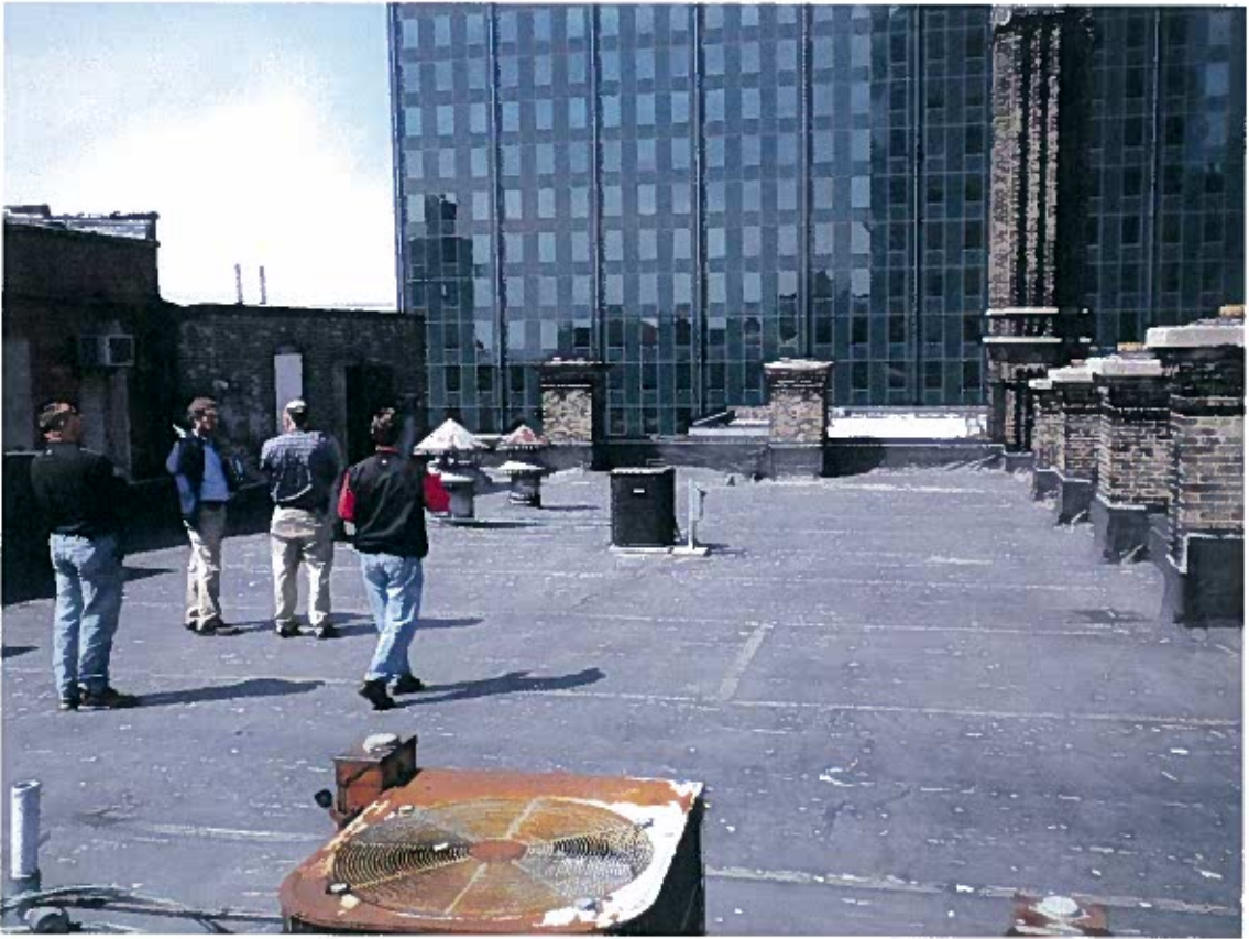
Photo 19: Roof, looking West
