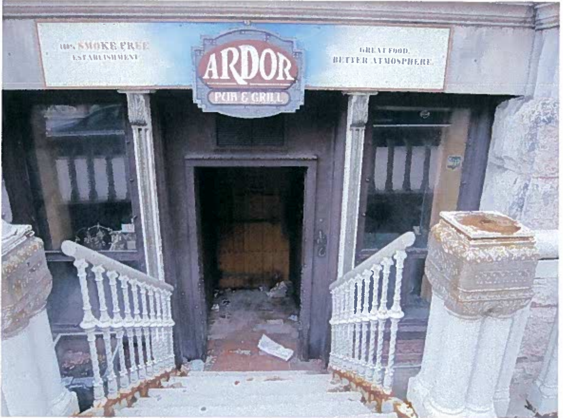
Photo 26: Ground Floor Broadway tenant entrance
