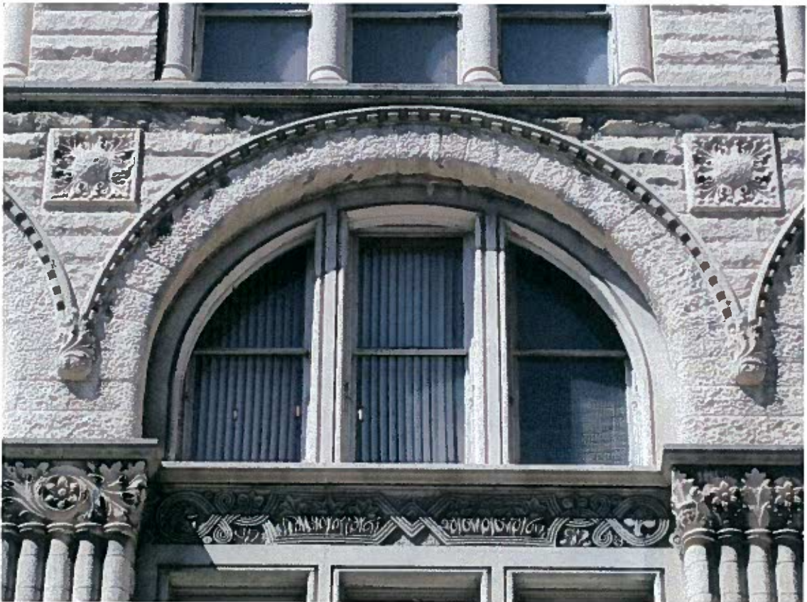
Photo 14: Fourth Floor window detail
