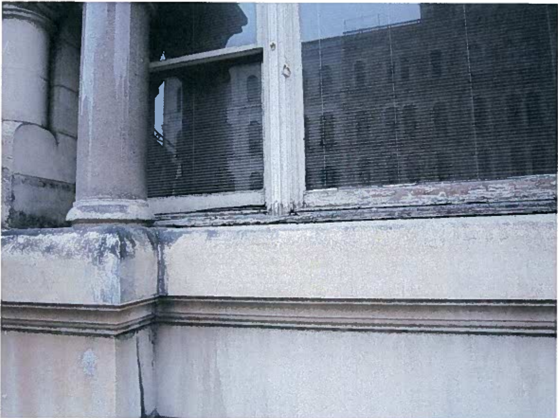
Photo 20: Typical window condition
