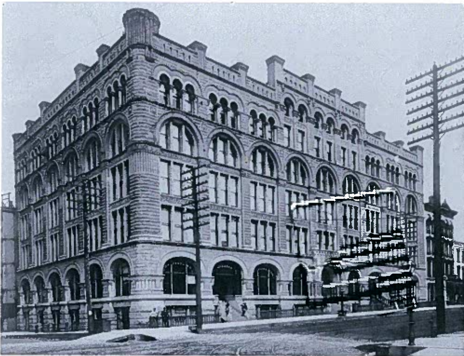
Photo 22: Corner of E. Michigan St. and Broadway, c. 1895
