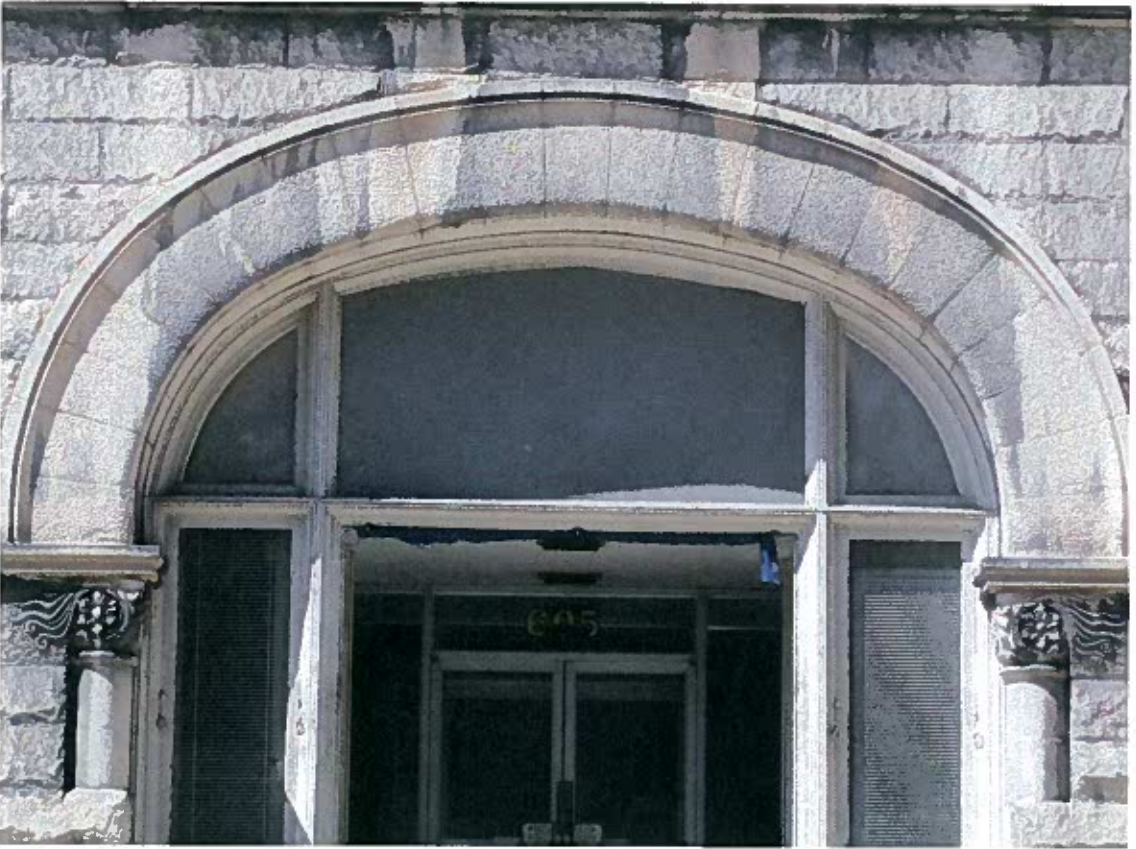
Photo 16: First Floor window detail
