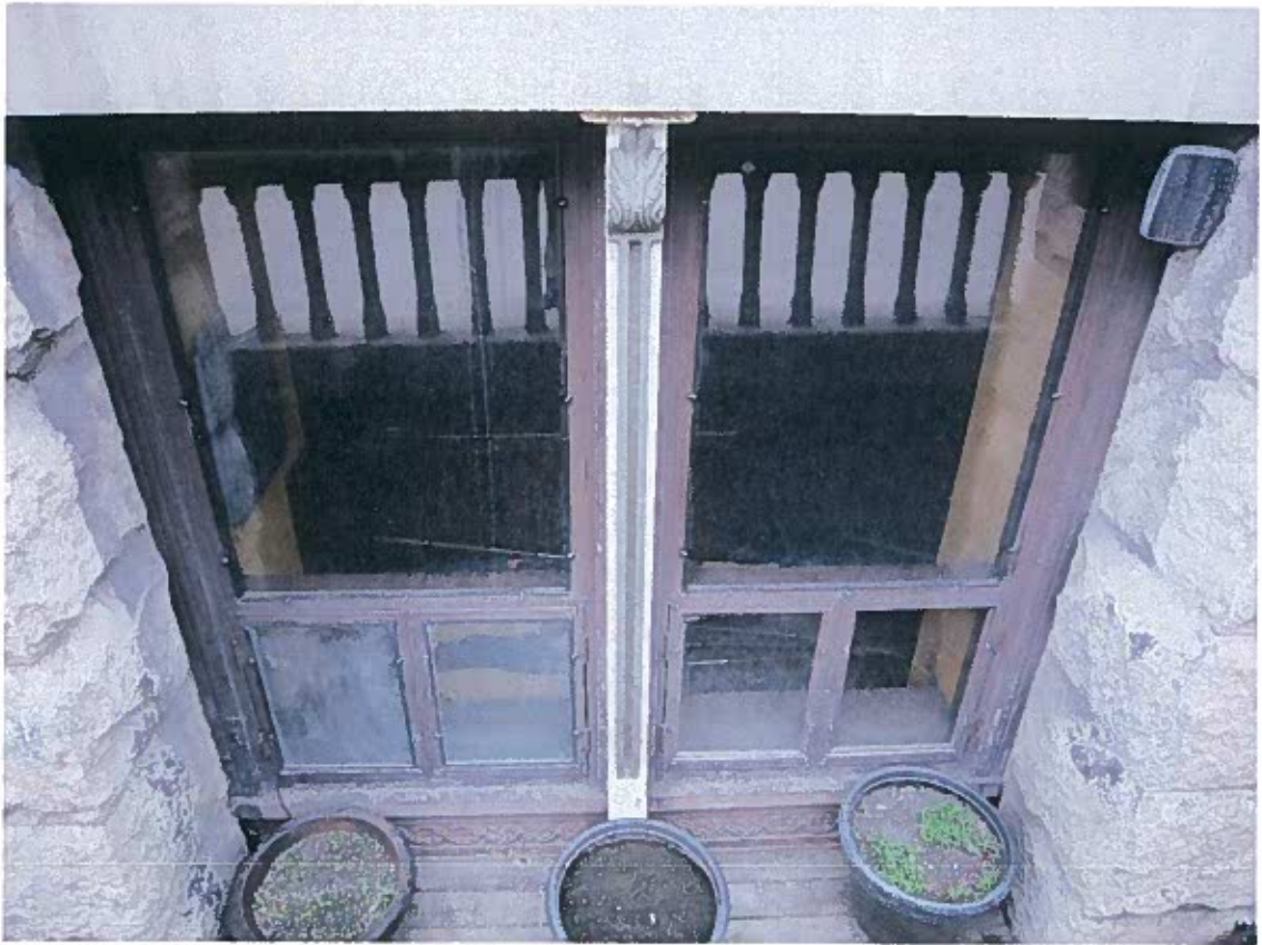
Photo 17: Ground Floor window detail
