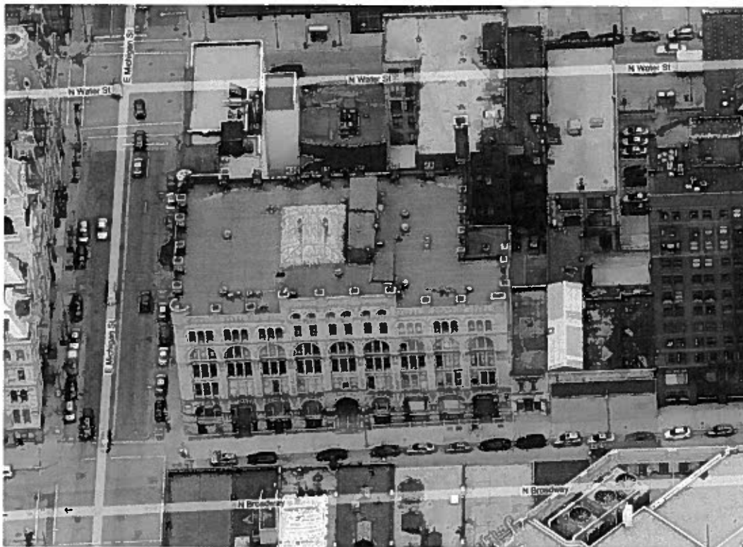
Photo 2: Aerial Looking West
