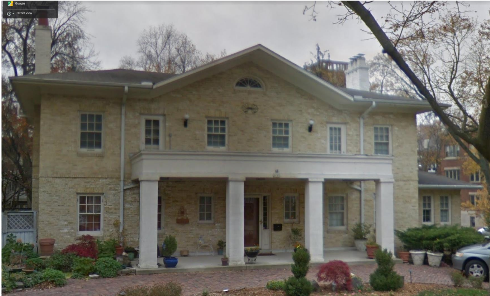
Subject house with present three-tab, dark gray shingles.
