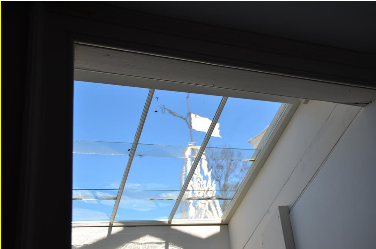
Skylight on 3 rd floor at Monticello
