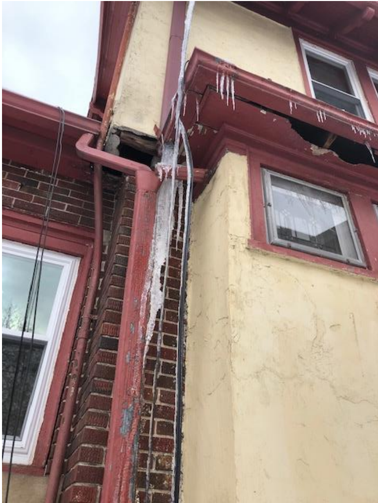
Typical soffit damage and overview of property
