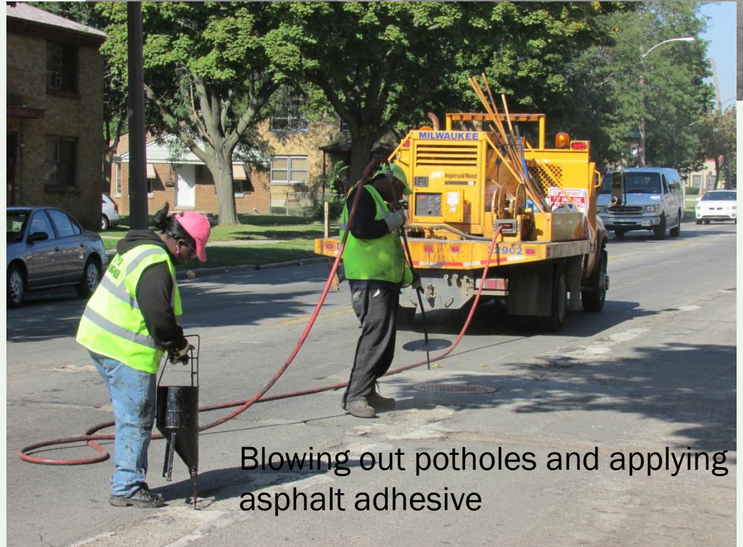
Pothole filling and patching
