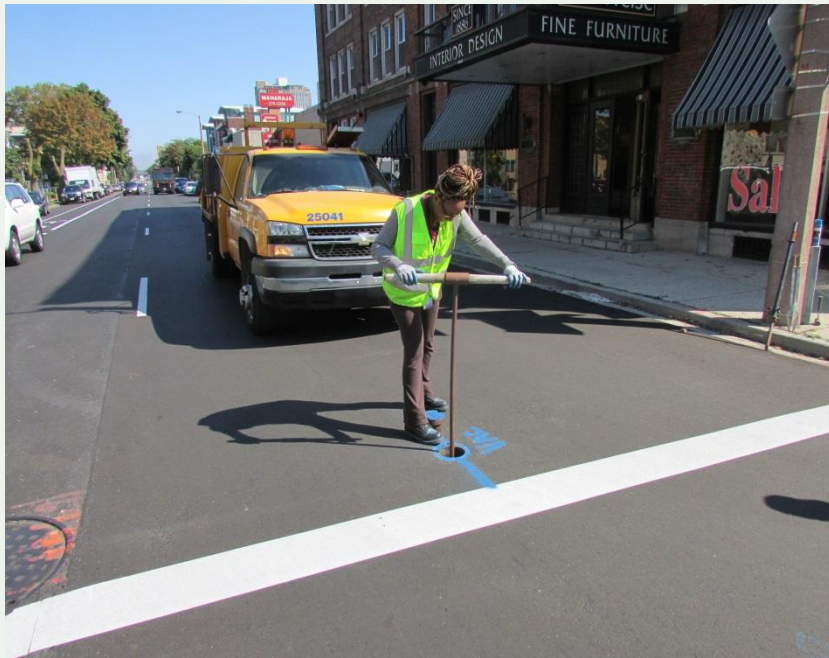
Exercising a water main valve
