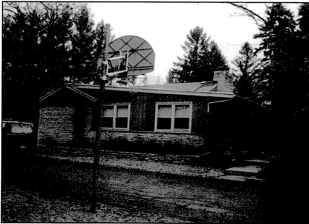
3031 S. ROOT RIVER PARKWAY EXTERIOR - SOUTHSIDE
