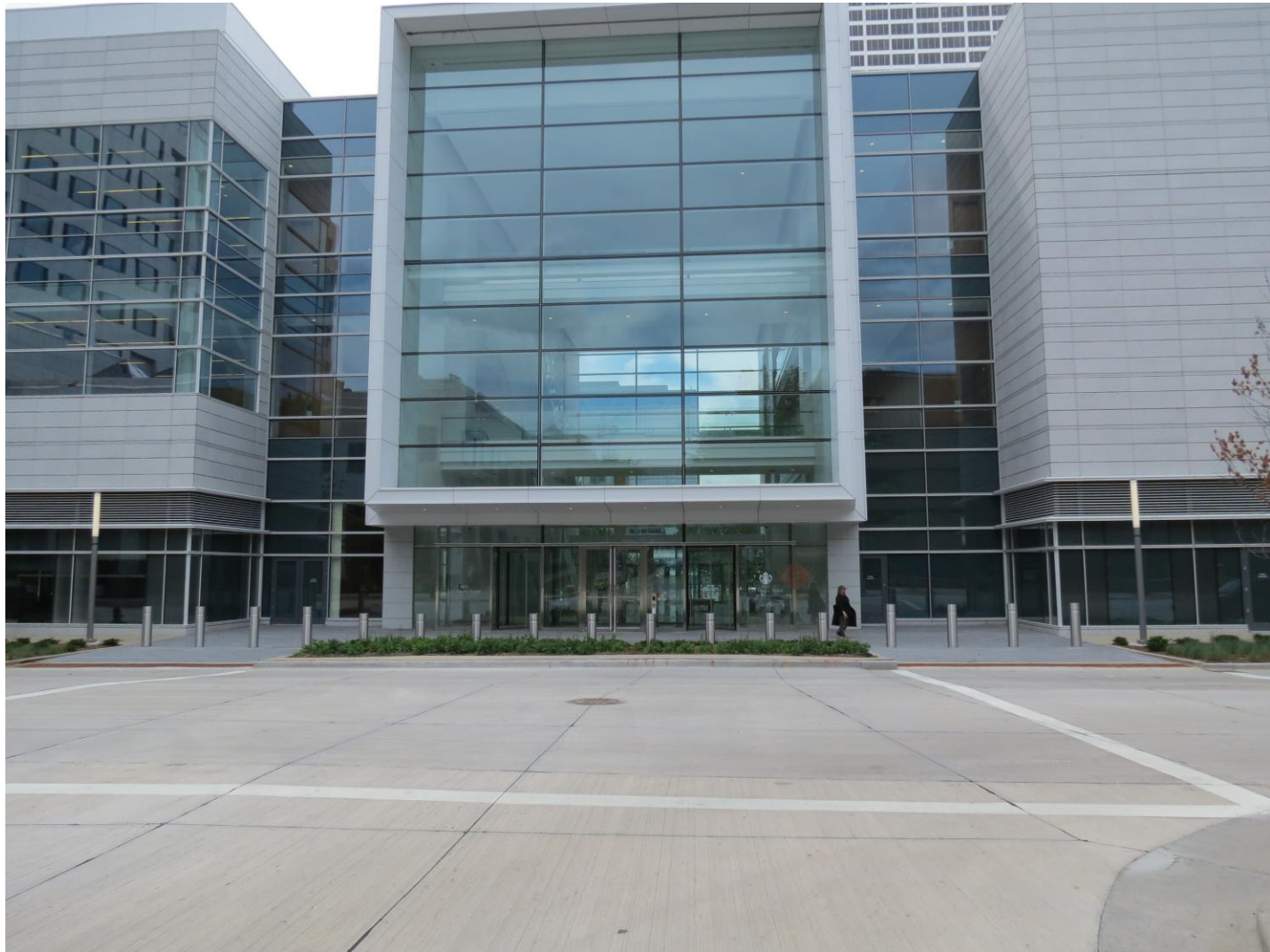
CCF 140507 Northwestern Mutual Life Insurance Company 8-9-2017 Looking south across East Mason Street towards the main building entrance located at North Cass Street. There are bollards, pavers, and private light fixtures at this location.
