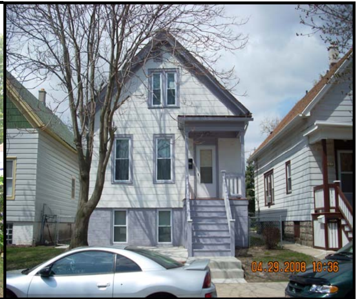
1519 S. 20 th Street – "After"
