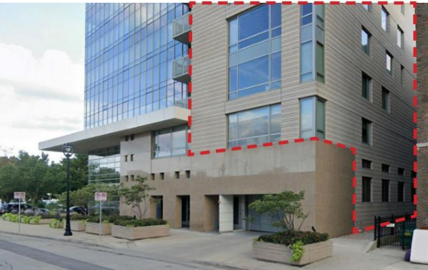
Precast Panel used in Kilbourn Tower
