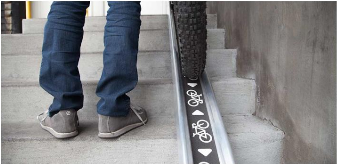
Bicycle Access Ramp Example
