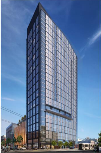
333 N. Water Street Milwaukee (under construction)
