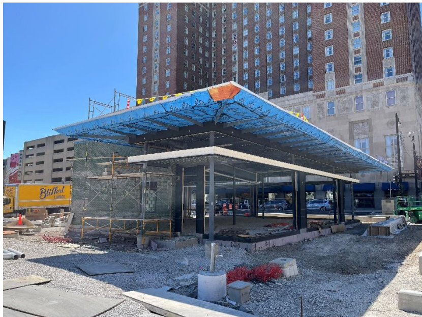
Photo of the Building, looking west
